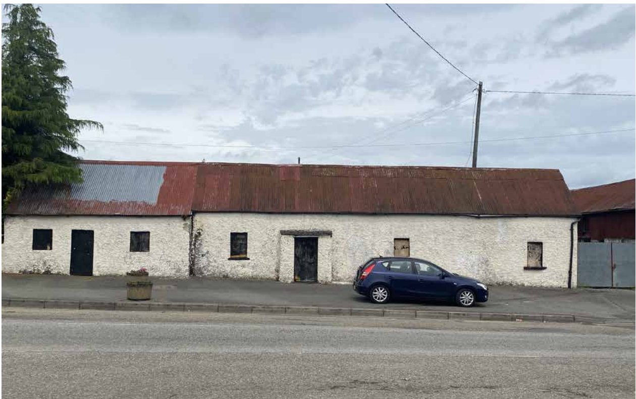
Figure 38 - Vacant historic cottages, Irishtown
