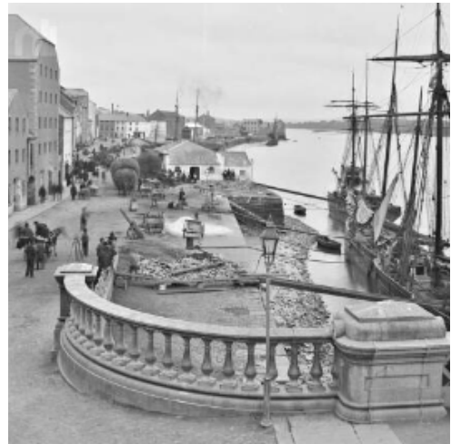
Figure 17 - Curved end of the new bridge with view down The Quay
