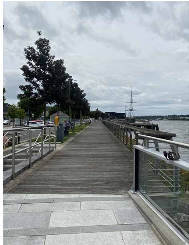
Figure 57 - View along the boardwalk with historic Quay Wall visible to right
