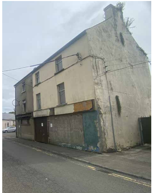
Figure 43 - Derelict building, Priory Street
