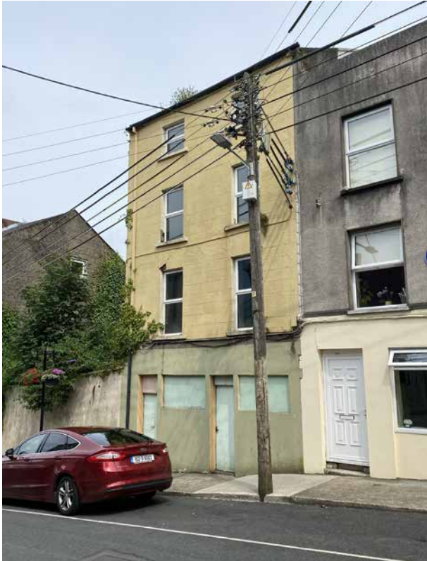
Figure 59 - Vacancy at ground floor and mass of electricity wires
