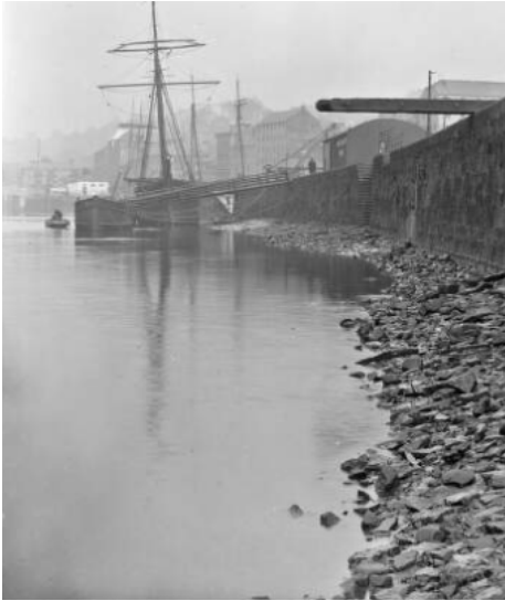
Figure 21 - Berth for ships with Quay wall visible, Oct 1924
