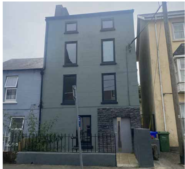
Figure 62 - Inappropriate alteration of historic house that fundamentally changes its character
