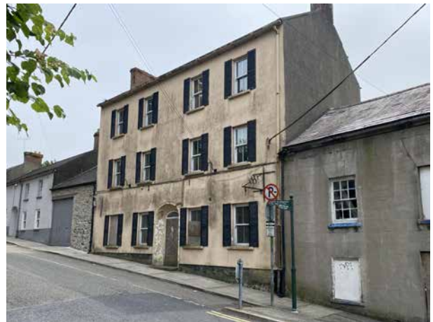
Figure 42 - Vacant houses, Mary Street Upper and corner of Bewley Street
