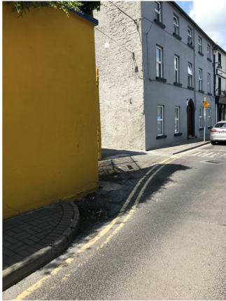
Narrow and discontinued footpaths, often without dished kerbs and hardly any tactile paving for universal access while bin refuge blocks access in many locations
