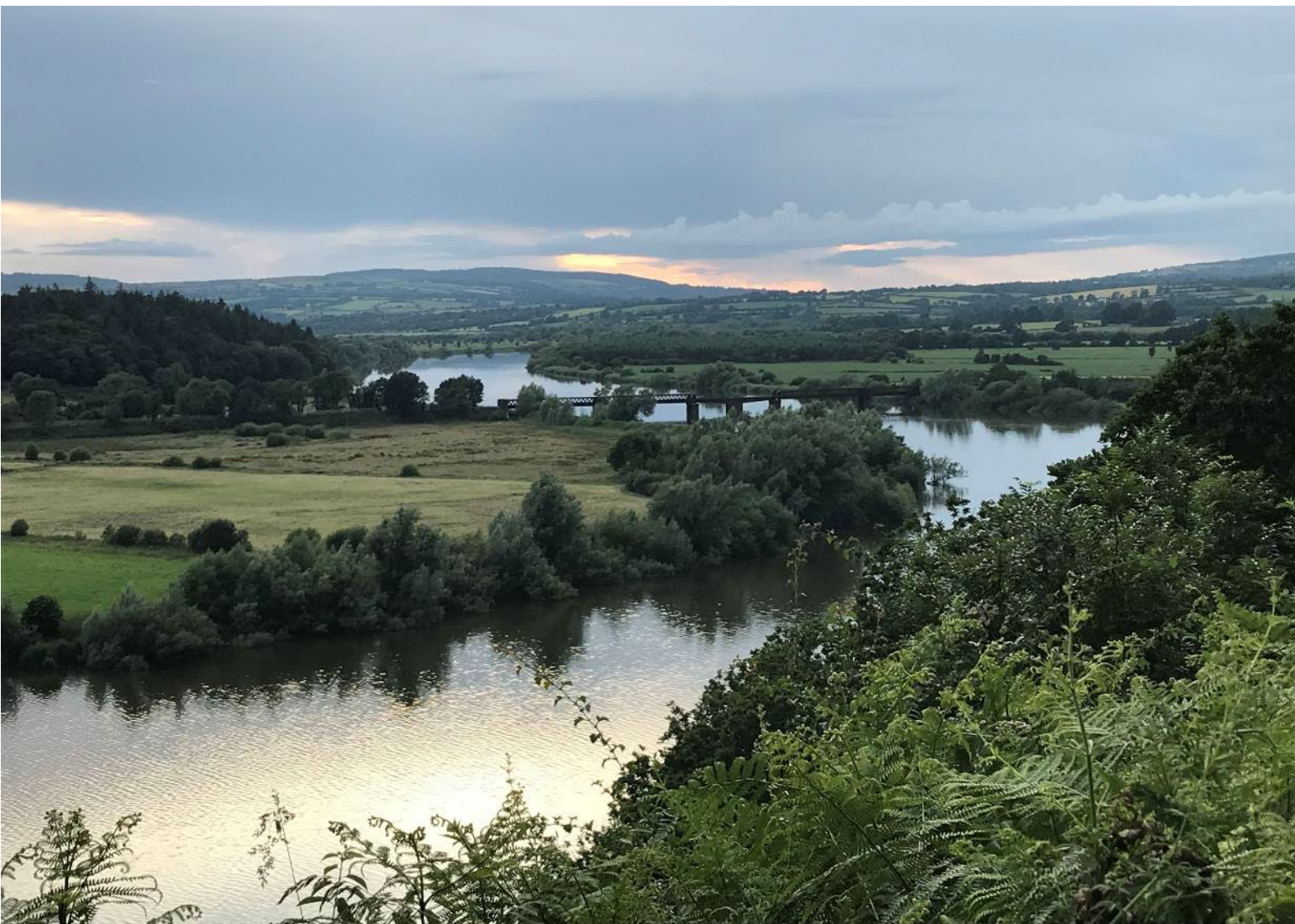
Red Bridge across the River Barrow, forming a section of the Greenway loop for New Ross
