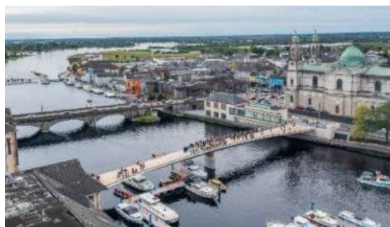
Athlone New Greenway Bridge
