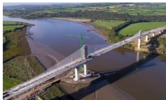
New Ross Bypass
