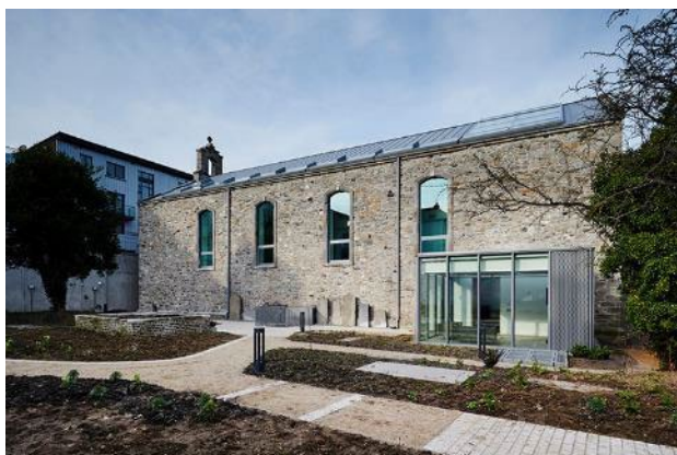
St Luke's Church, Dublin was refurbished and converted to offices.
