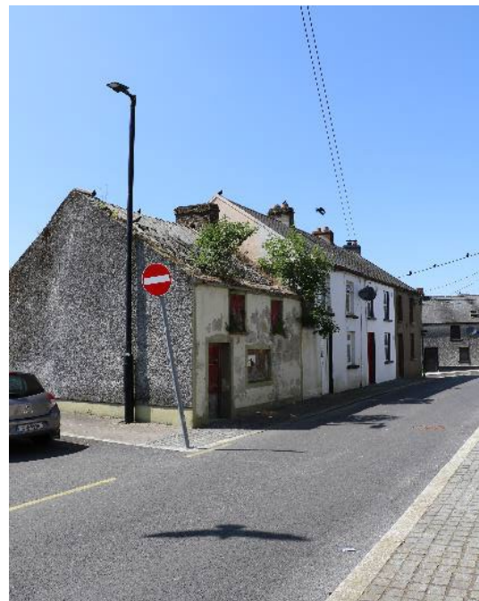
Derelict terraced townhouse
