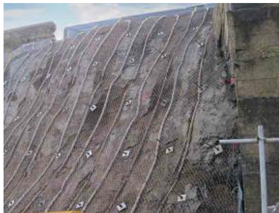
Figure 5-5: Typical Image of Cliff Stabilisation
