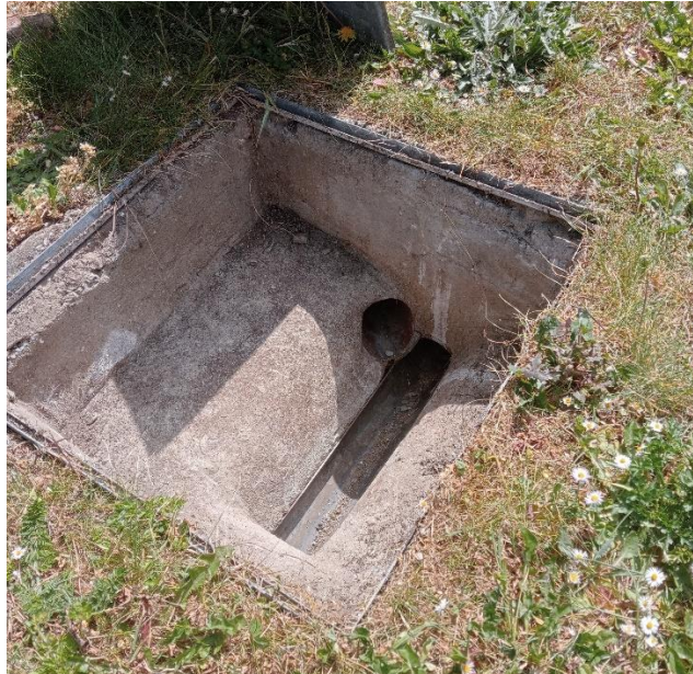
Figure 3-4: Existing Drainage Chamber/Channels (West of Zone 02)
