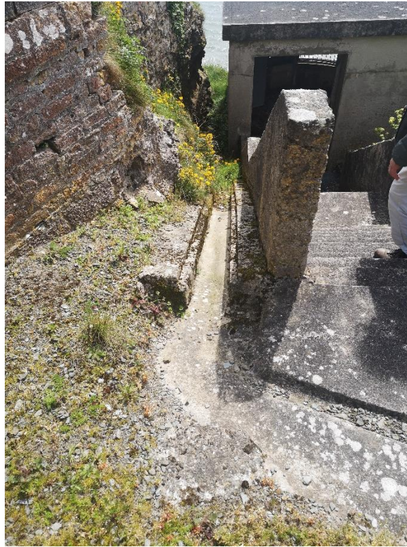
Figure 3-5: Existing Drainage Outlet Channel (South-west of Zone 02)
