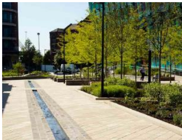
Figure 5-3: Typical Image of a Channel and Rill SuDS
