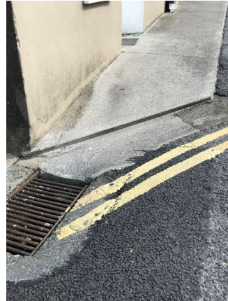
Narrow and discontinued footpaths, often without dished kerbs and hardly any tactile paving for universal access while bin refuge blocks access in many locations
