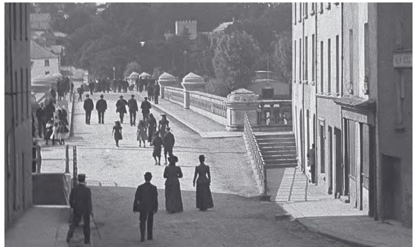
Old Bridge looking west (demolished 1968) late 19 th century
