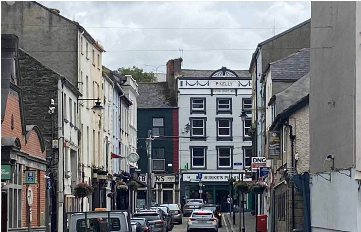
Figure 73 - View up Charles Street from The Quay to South Street
