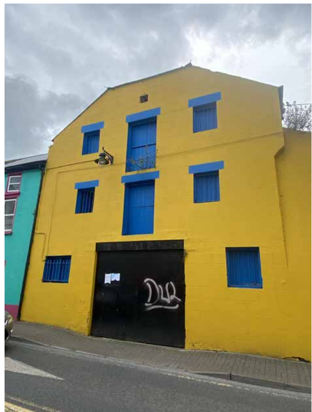
Figure 52 - Recently painted building, Sugar House Lane
