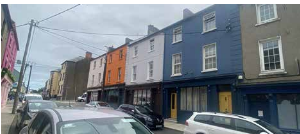
Figure 51 - Restored shopfronts, Priory Street
