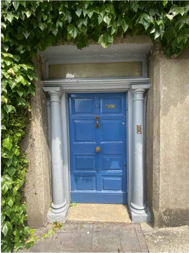
Figure 53 - Door, Bridge Street
