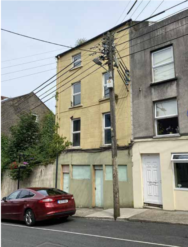
Figure 59 - Vacancy at ground floor and mass of electricity wires
