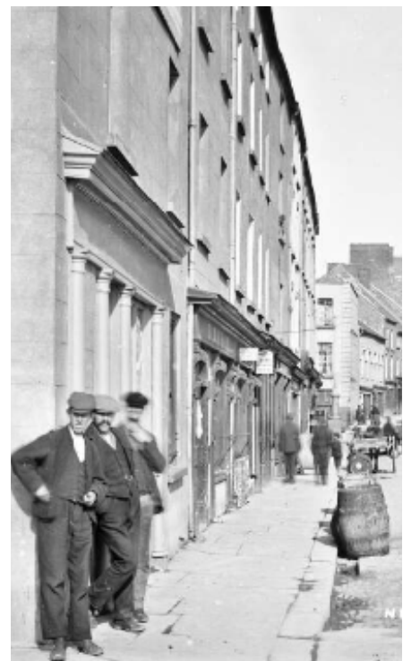
Figure 19 - Corner of The Quay & Quay Street
