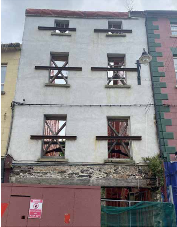
Figure 39 - Surviving facade, John Street
