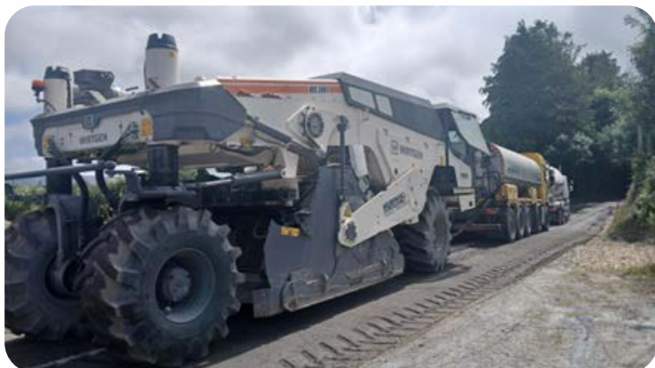
Road strengthening works underway on L-3009-3 near Glynn, Wexford BD, using road recycling methods.
