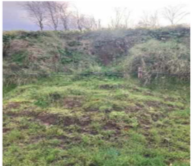
Figure 2.9: Embankment slippage
