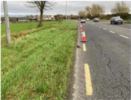
Figure 2.11: Longitudinal cracking in pavement adjacent embankment slippage
