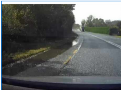
Figure 2.21: Ponding on hard shoulder
