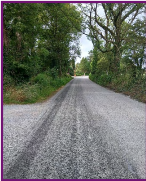
Surface Dressing underway at Rosslare MD, June 2026
