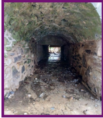
Works underway at Raheendarrig Bridge on the L-1003 at Clone West, Monamolin, Gorey-Kilmuckridge MD
