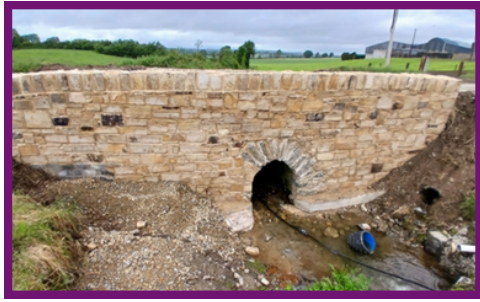
Ballintarton Bridge / Culvert completed works – Bridge Rehab works. Rosslare MD
