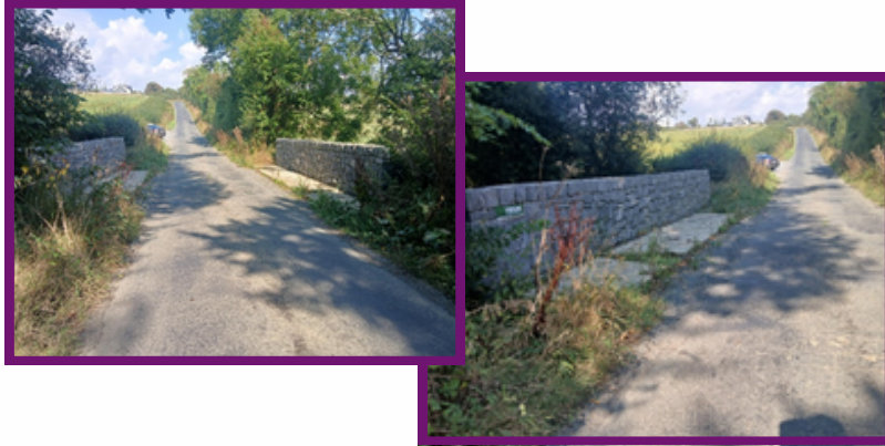
Restoration works at Taulaught Bridge, St Kearns – under the Climate Change Adaptation and Resilience Works. New Ross MD.
