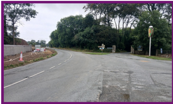
L4043 Tintern – Safety Improvement Works underway – improving sightlines at entrance to Tintern Abbey. New Ross MD.
