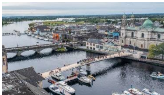
Athlone New Greenway Bridge
