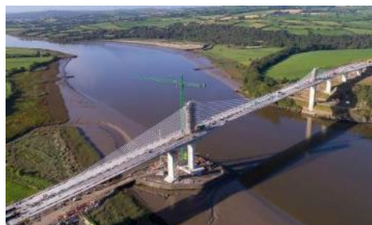
New Ross Bypass
