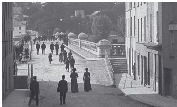
New Ross Historic Bridge
