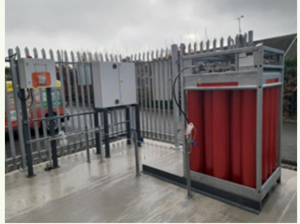
Pictured BioGas installation, gas storage cylinders and a decompression unit in secure compound
