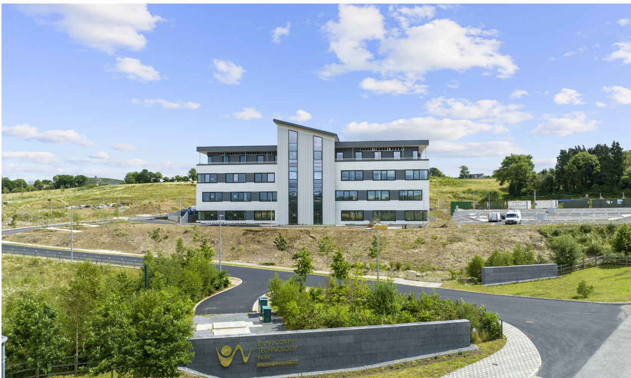
The energy efficient office building in Enniscorthy Technology Park (Wexford County Council)
