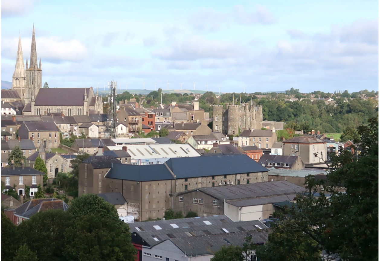
A view of Enniscorthy (Wexford County Council)
