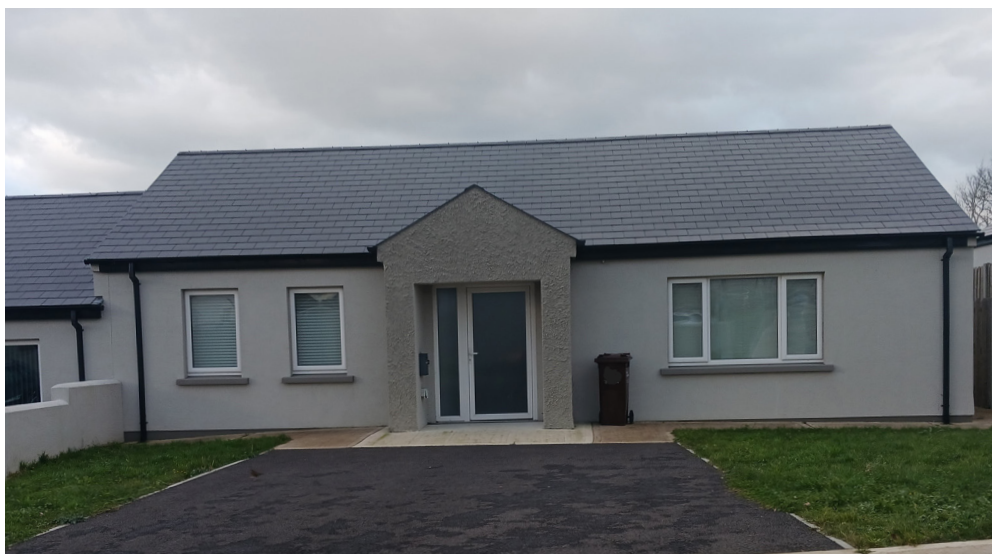
Droichead Carley, Enniscorthy, all new social housing built to Nearly Zero Energy Build standard.
