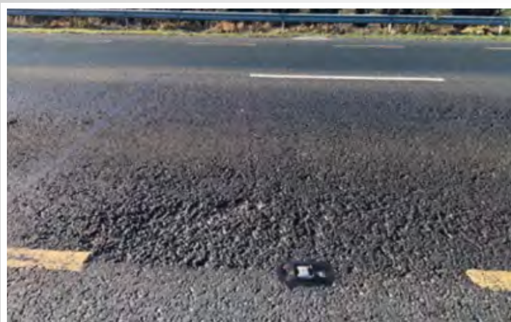
N11 Oilgate Village Pavement Repair. Works Completed
