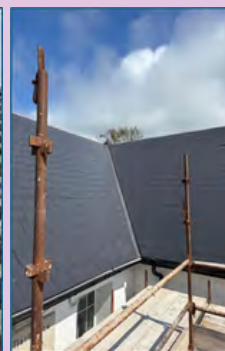
Kilrane Rosslare Harbour Community Centre - roof repairs
