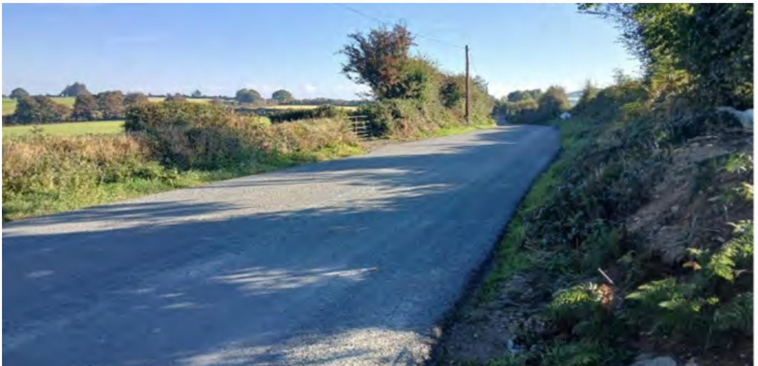
Recent RI Strengthening Works at Kellystown Road, New Ross MD
