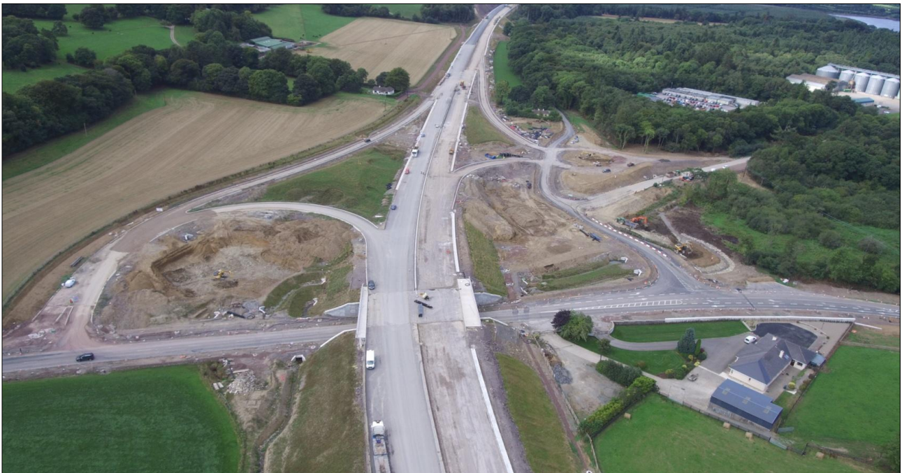
6. R733 Junction – Formation of slip roads in progress, construction of roundabout at Stokestown Road (centre right)
