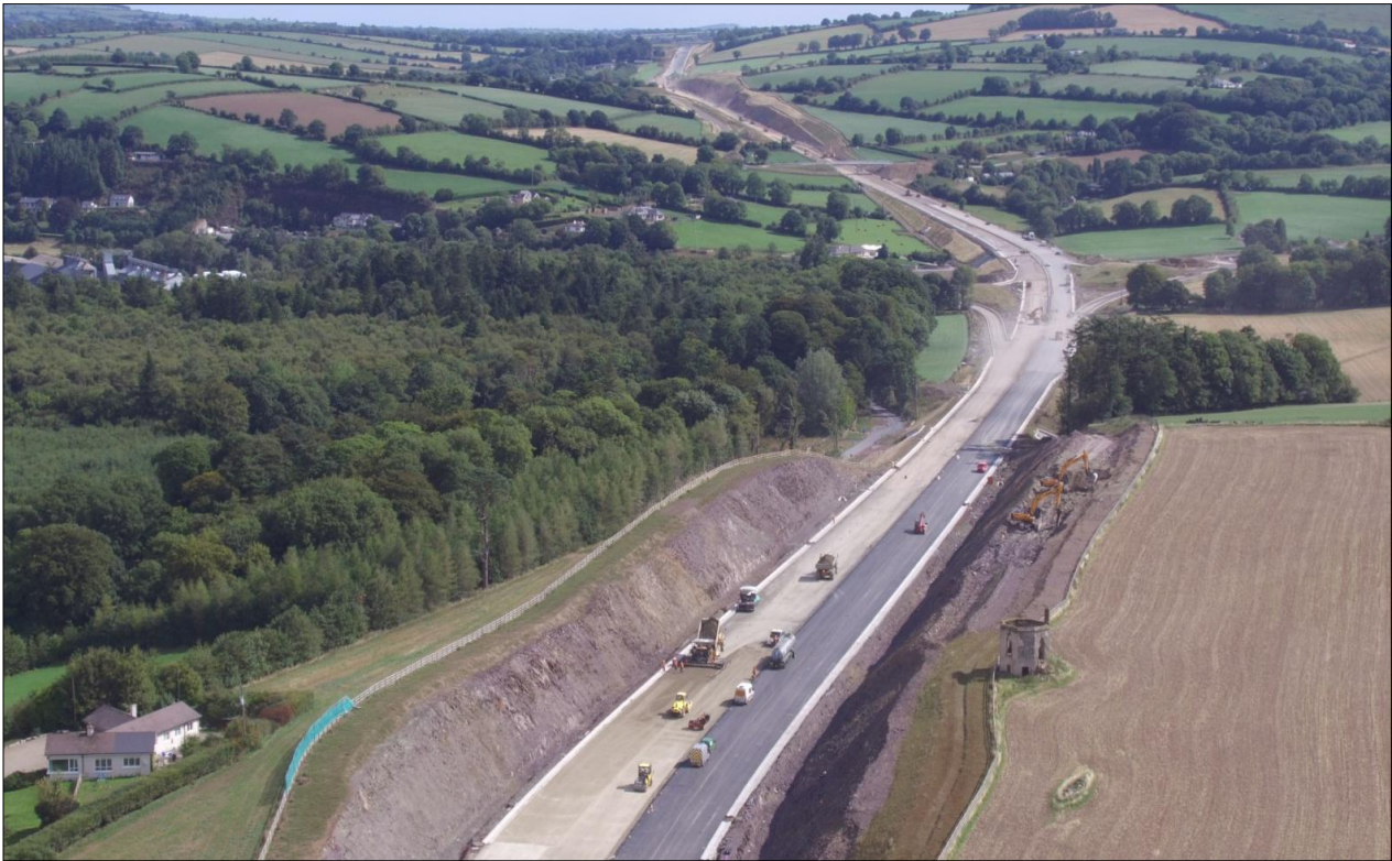
5. Cut 3 at Stokestown & Landscape – Earthworks and pavement works in progress.
