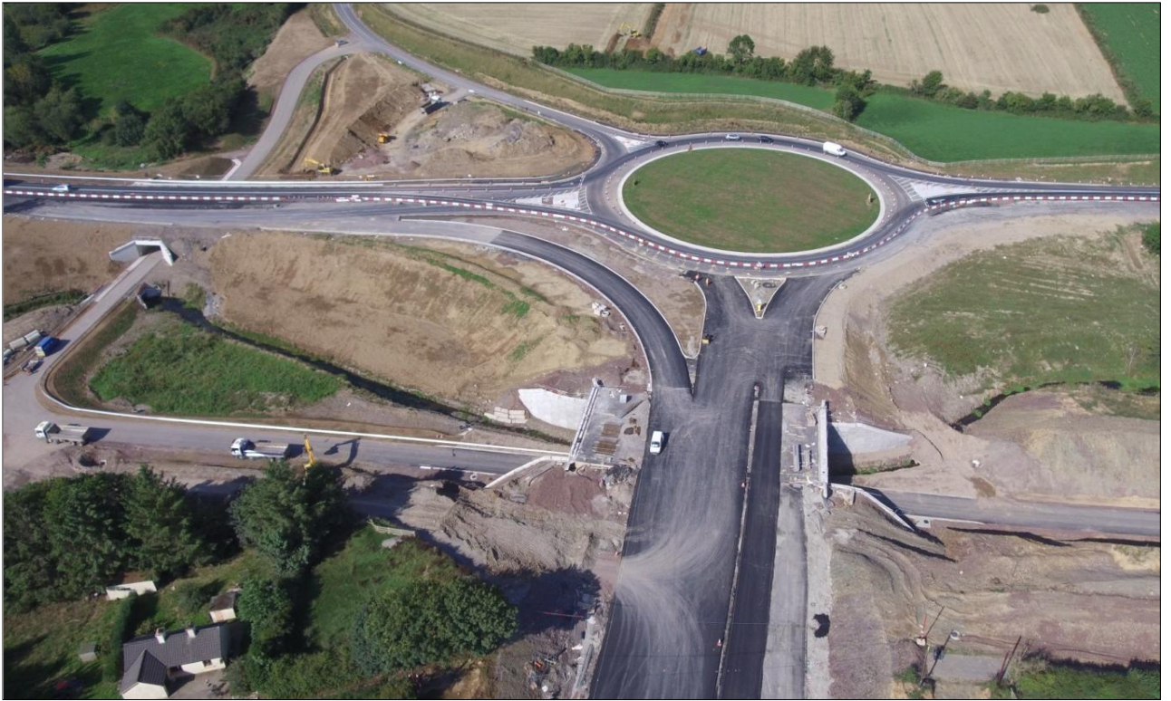
1. Glenmore Roundabout open under temporary traffic management. Bypass tie in to roundabout under construction in the foreground. Bridges and road realignments under construction in the foreground and left to facilitate local road access.
