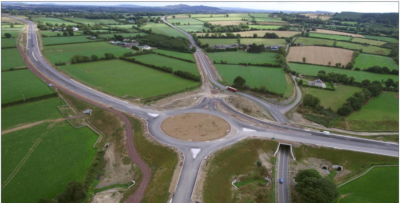
7. N25 Ballymacar Roundabout - Final surfacing works in and tie-ins to existing road to be completed.
