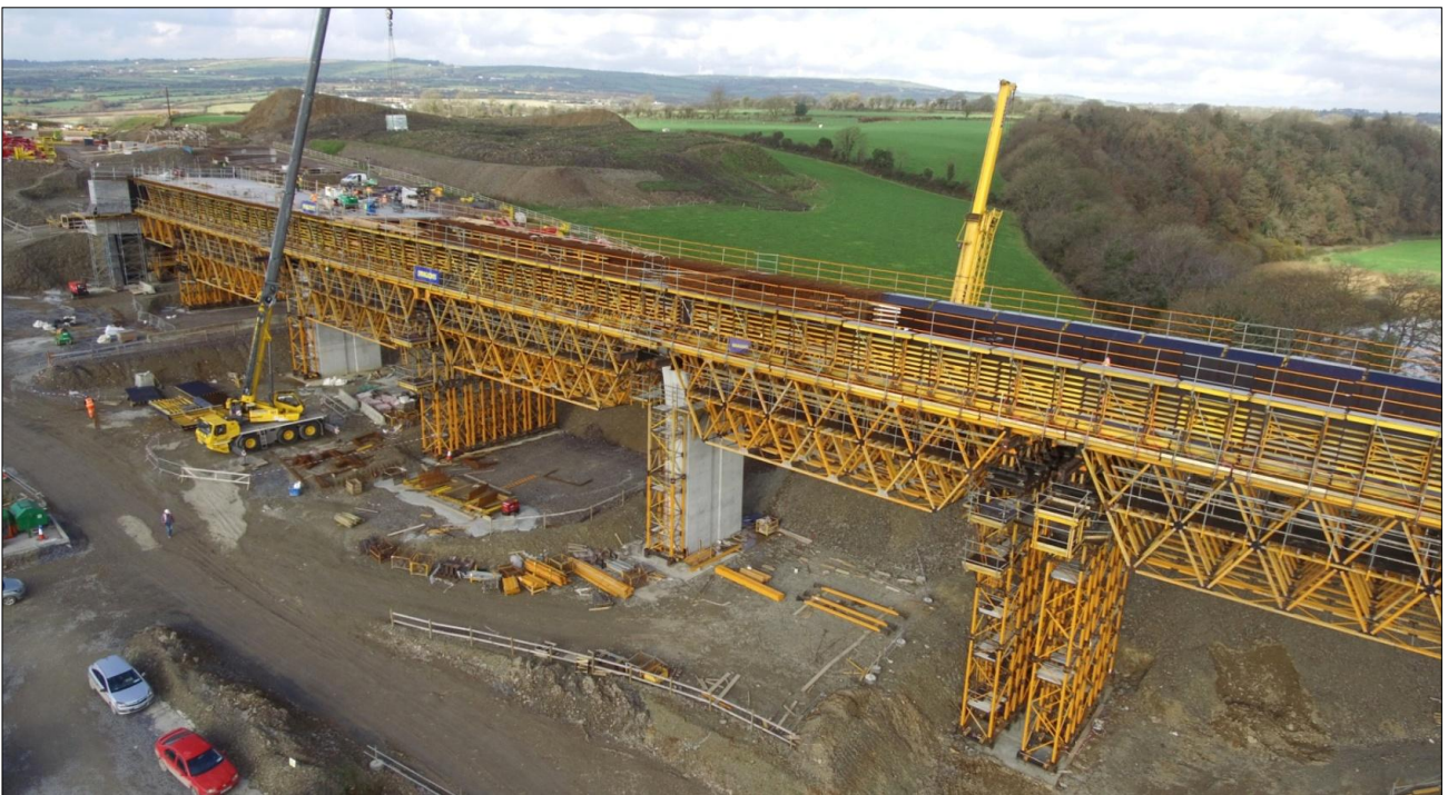
1. Barrow Bridge – Deck falsework in place for approach spans 2 & 3 at Pink Rock to bottom left of photo. River pier in background.
