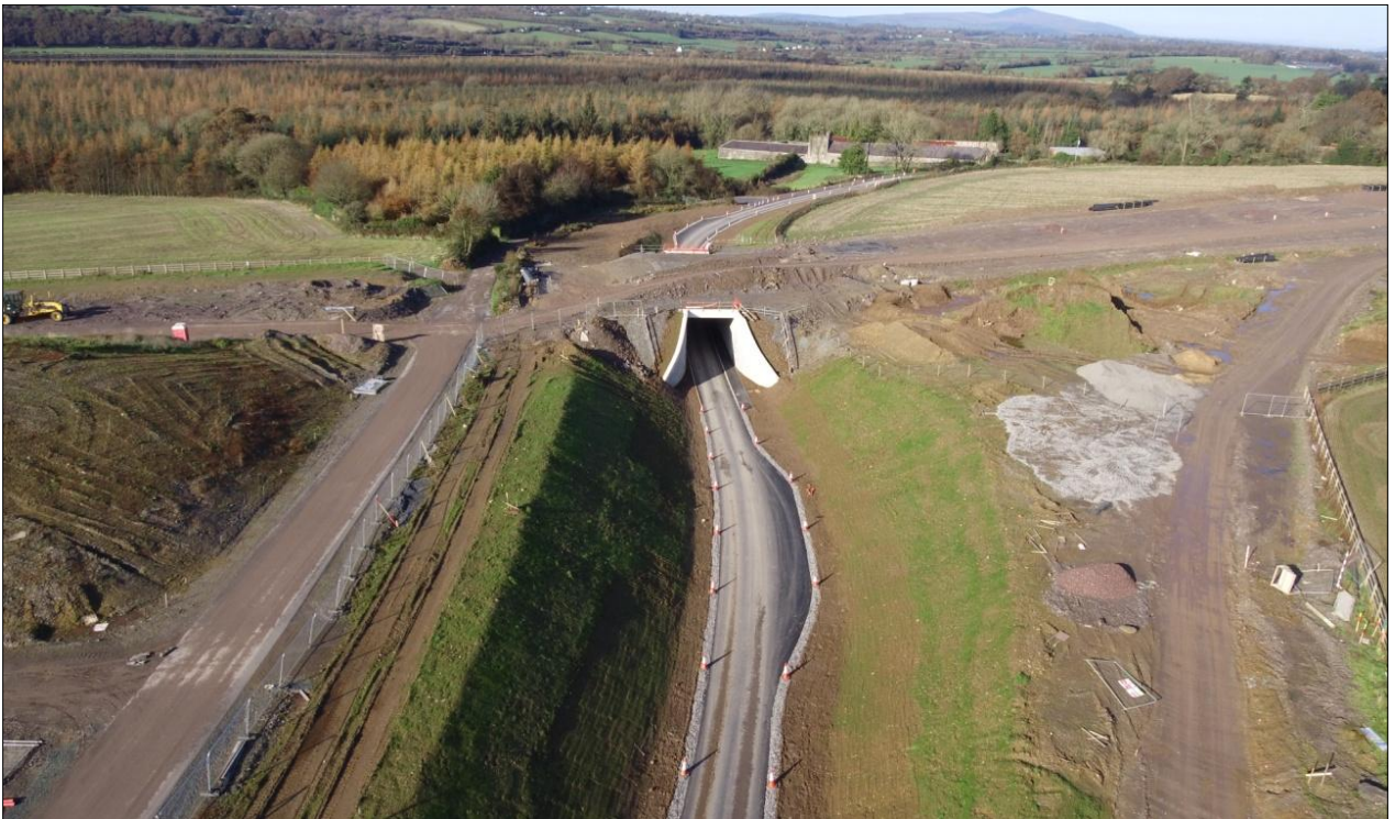
4. Stokestown Road bridge and new alignment with passing bays.
