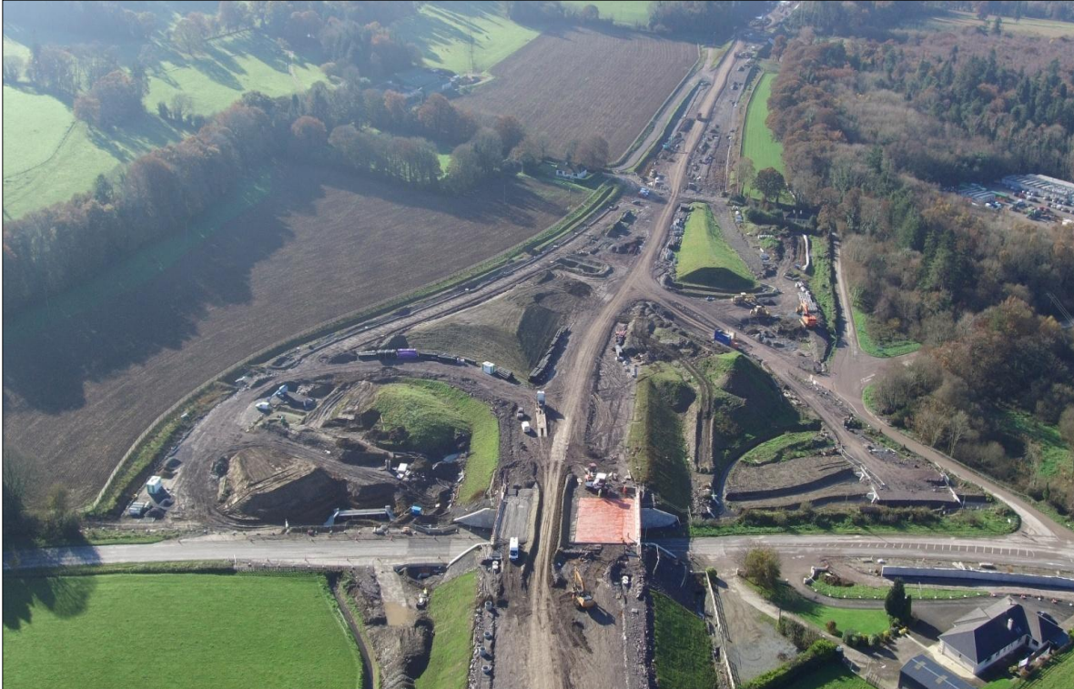
7. R733 grade separated junction taking shape.
