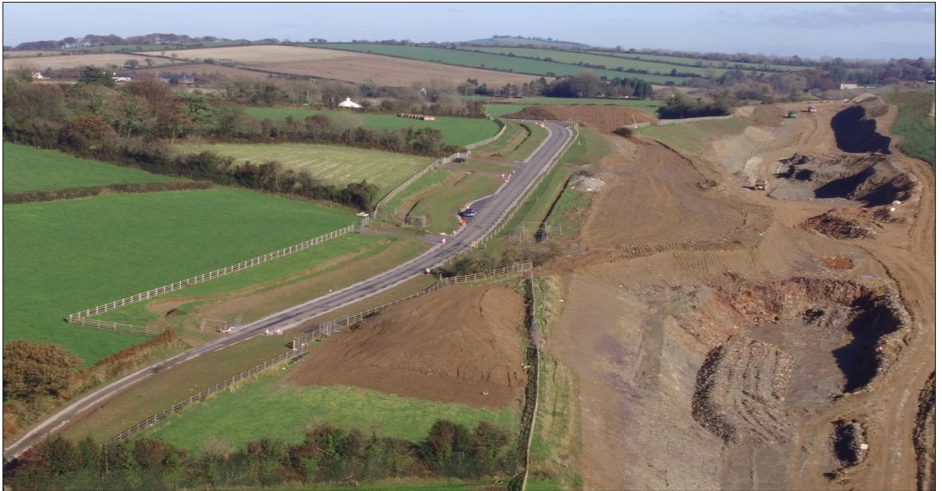
6. Local road realignment at Camlin – new road realignment to left of picture (with passing bays), earthworks to right (rock blasting site).
