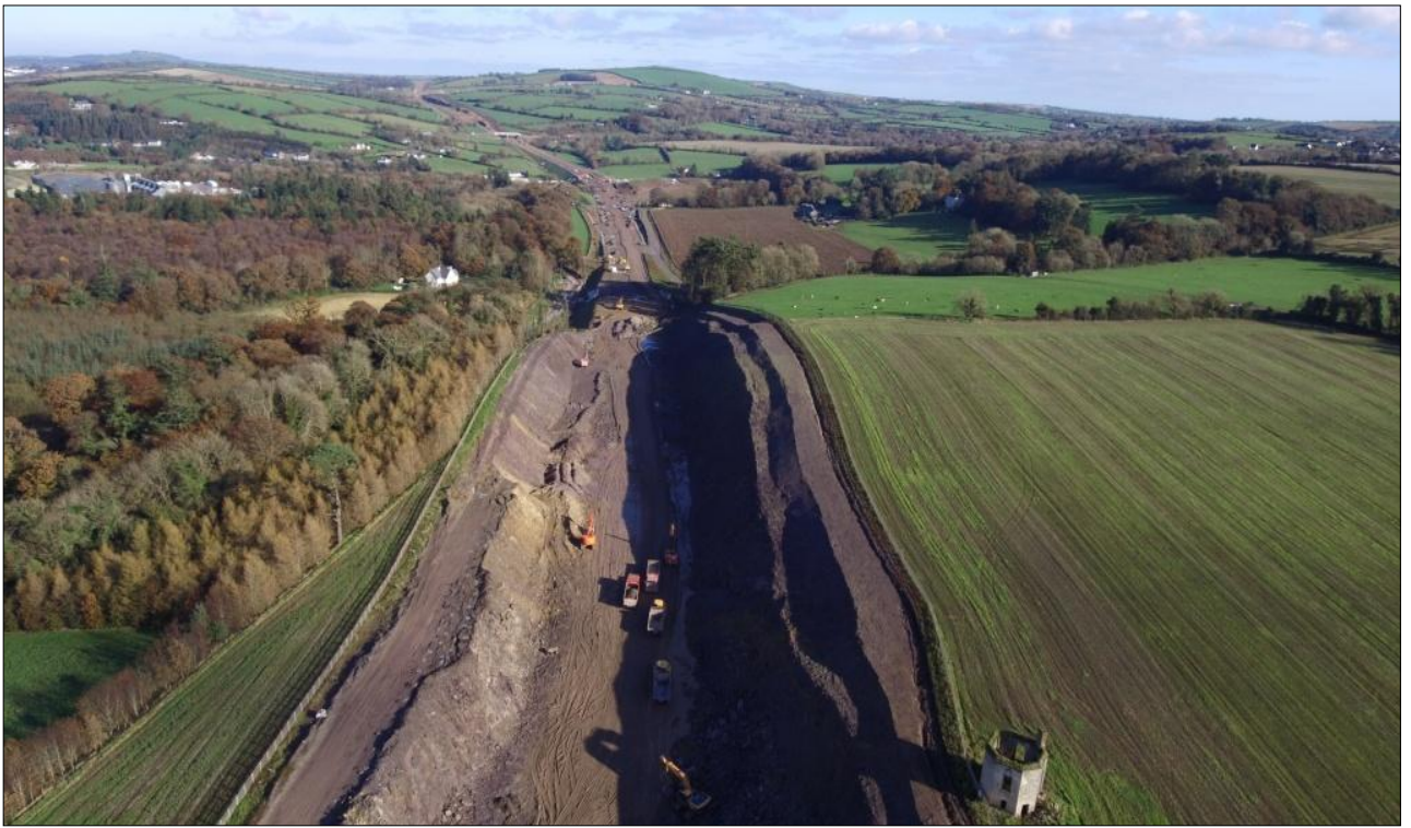
5. Earthworks at Stokestown (rock blasting site).
