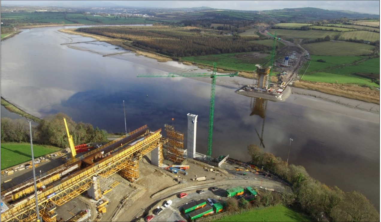
1. Barrow Bridge – Deck falsework in place for approach spans 2 & 3 at Pink Rock to bottom left of photo. River pier in background.
