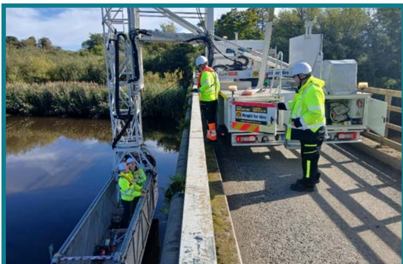
Edermine Bridge, Detailed Structural Investigation Works underway. Enniscorthy MD
