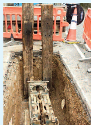
Pipe bursting trenchless technology - Summer Hill, Wexford
