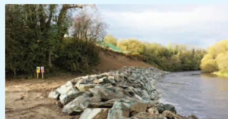
Slope Stabilisation works Bunclody WWTW - After
