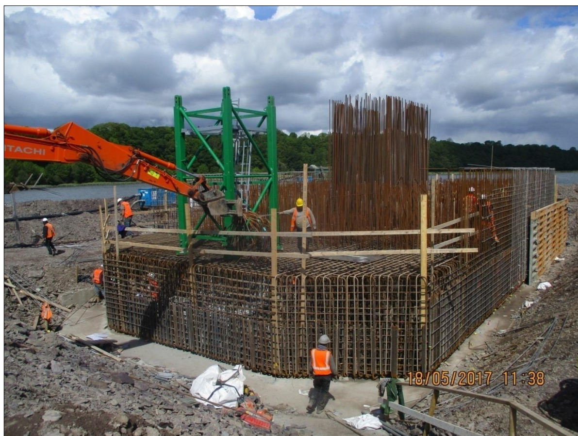
5. Barrow Bridge - Pier 4 steel fixing for base and plinth
