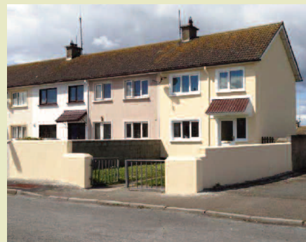
After Improvement works
