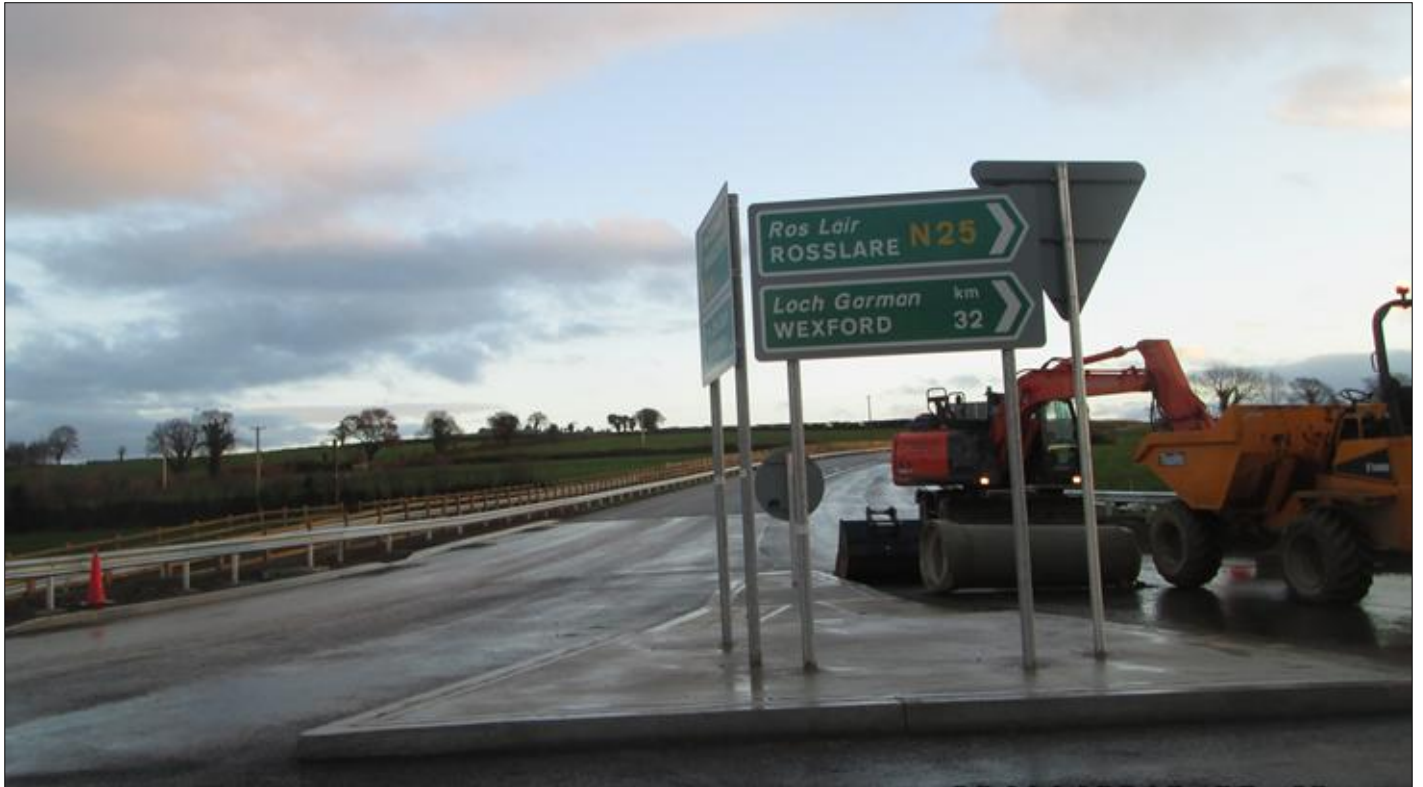
5. N25 Ballymacar Roundabout – Erection of signage.
