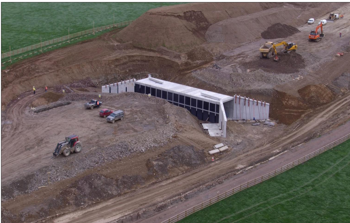
accommodation underpass under construction
