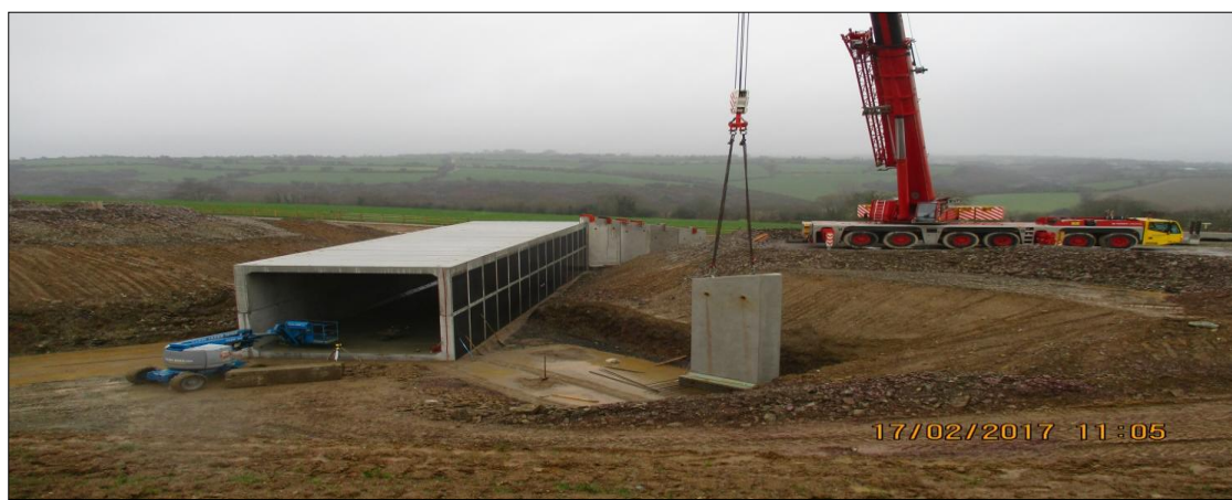
6. Beam Lift operations under traffic management at R733 Underbridge
