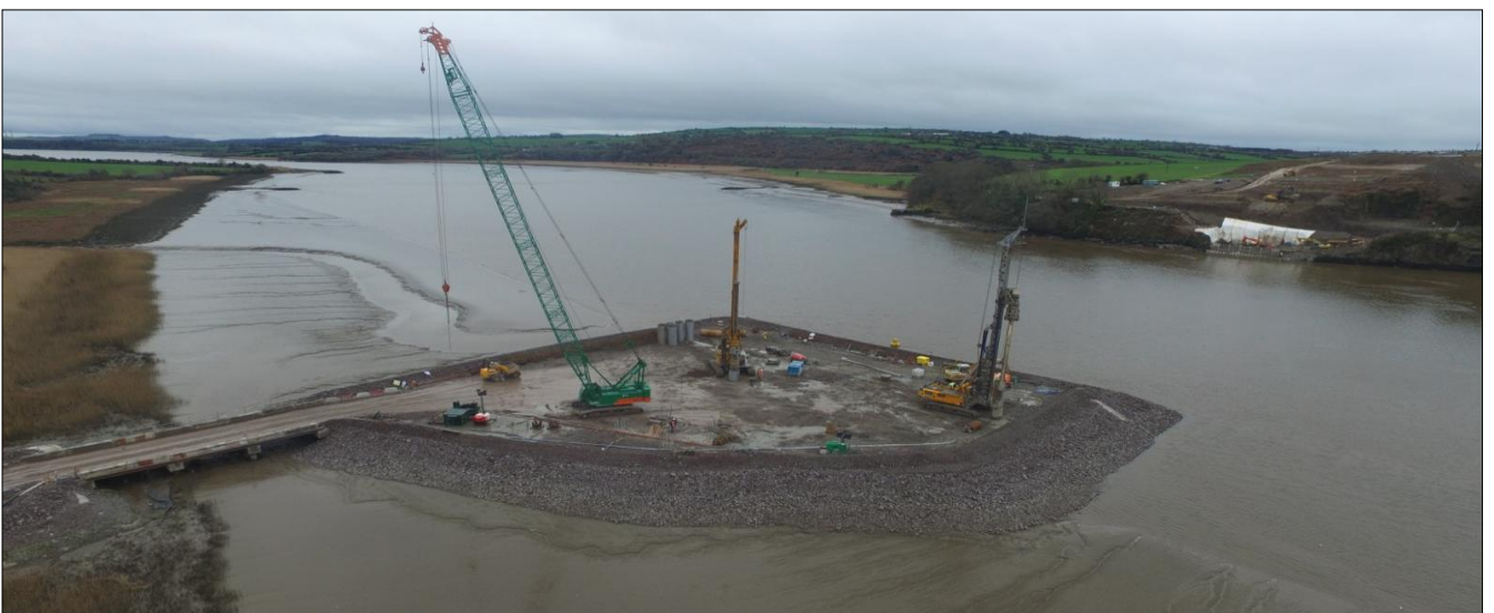
1. Barrow Bridge - Preparatory works for pier foundations on Co. Kilkenny side in foreground with Pier 4 in background.
