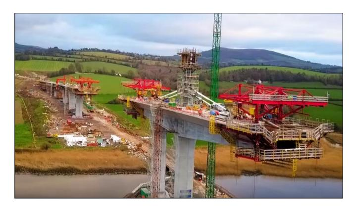
1. Rose Fitzgerald Kennedy Bridge – Construction of pylon tower and installation of cables at Pier 4 in foreground. Pier 5 and approach spans on Wexford side in background.
