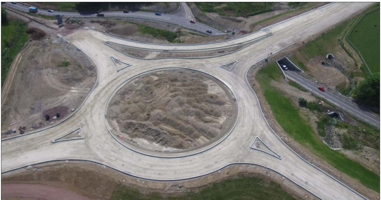
6. N25 Ballymacar Roundabout – kerbing and pavement foundations complete
