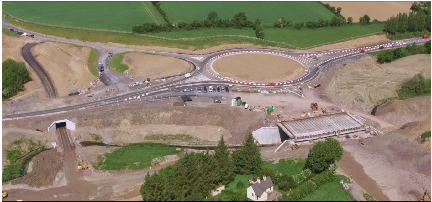
1. Glenmore Roundabout fully open under temporary traffic management. Glenmore Road Underbridge to left, Ballyverneen Road Underbridge to bottom right providing grade separated access for local traffic.
