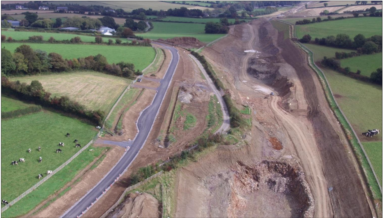
6. Earthworks at Stokestown (rock blasting site).
