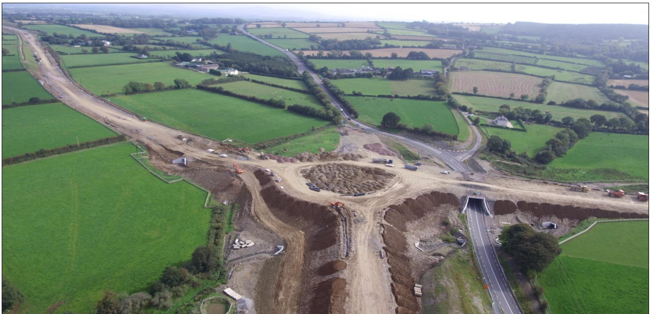
7. Local road realignment at Camlin – new road realignment to left of picture, old local road to centre, and bypass under construction to right.
