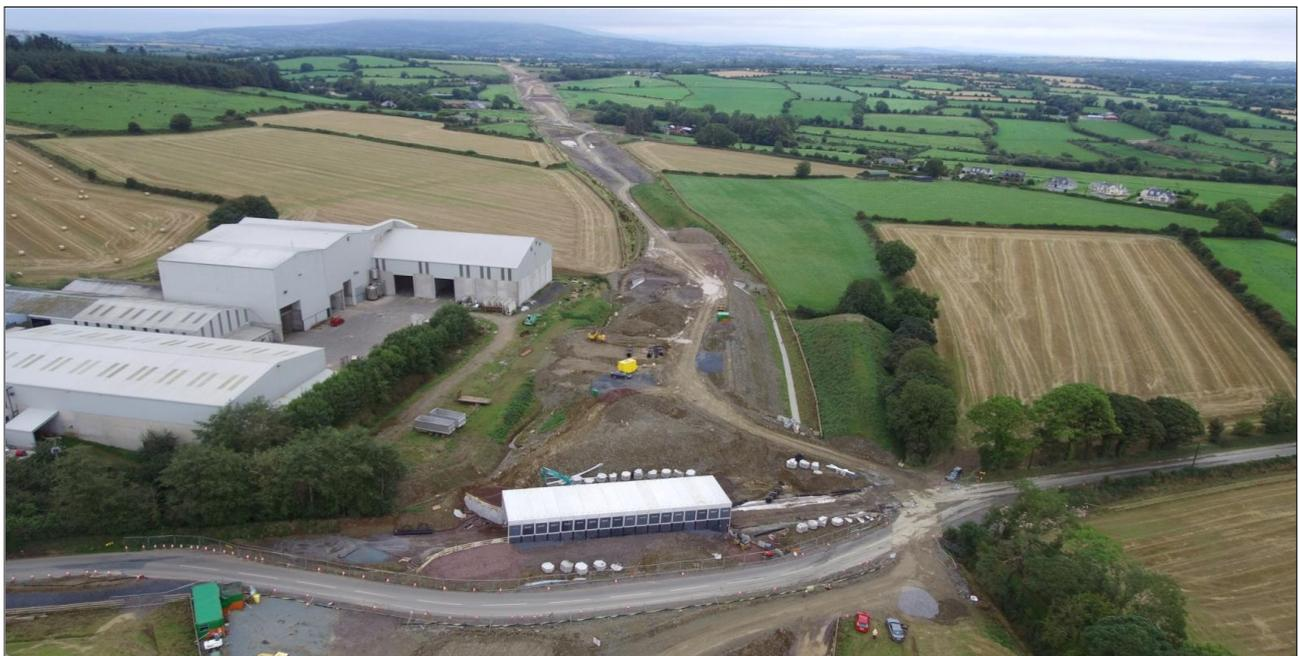
9. Ryleen Road Underbridge – an example of local road temporary diversion and traffic management around a road bridge construction site.
