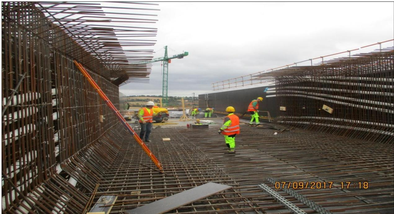
4. Barrow Bridge – Steel fixing in deck box for approach spans 1 & 2.
