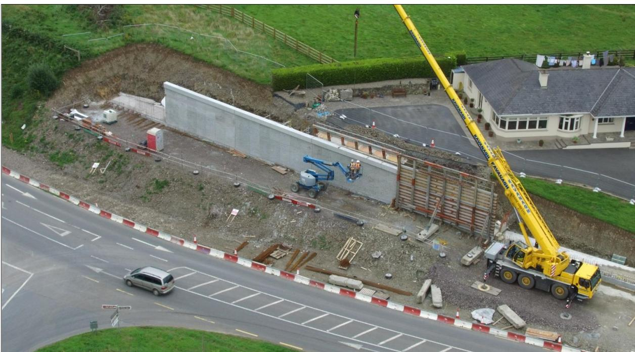
7. Construction of retaining wall to accommodate road realignment at R733
