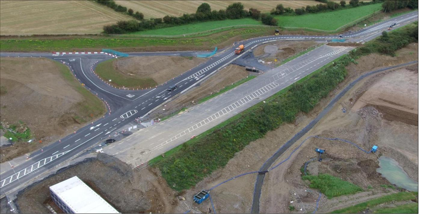
1. Temporary diversion and traffic management at N25 Glenmore for construction of roundabout and road underpass (underpass installation at bottom of photo).
