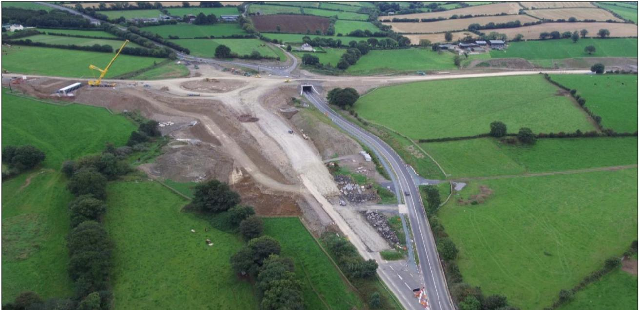
8. Temporary diversion route at Ballymacar for construction of online roundabout.
