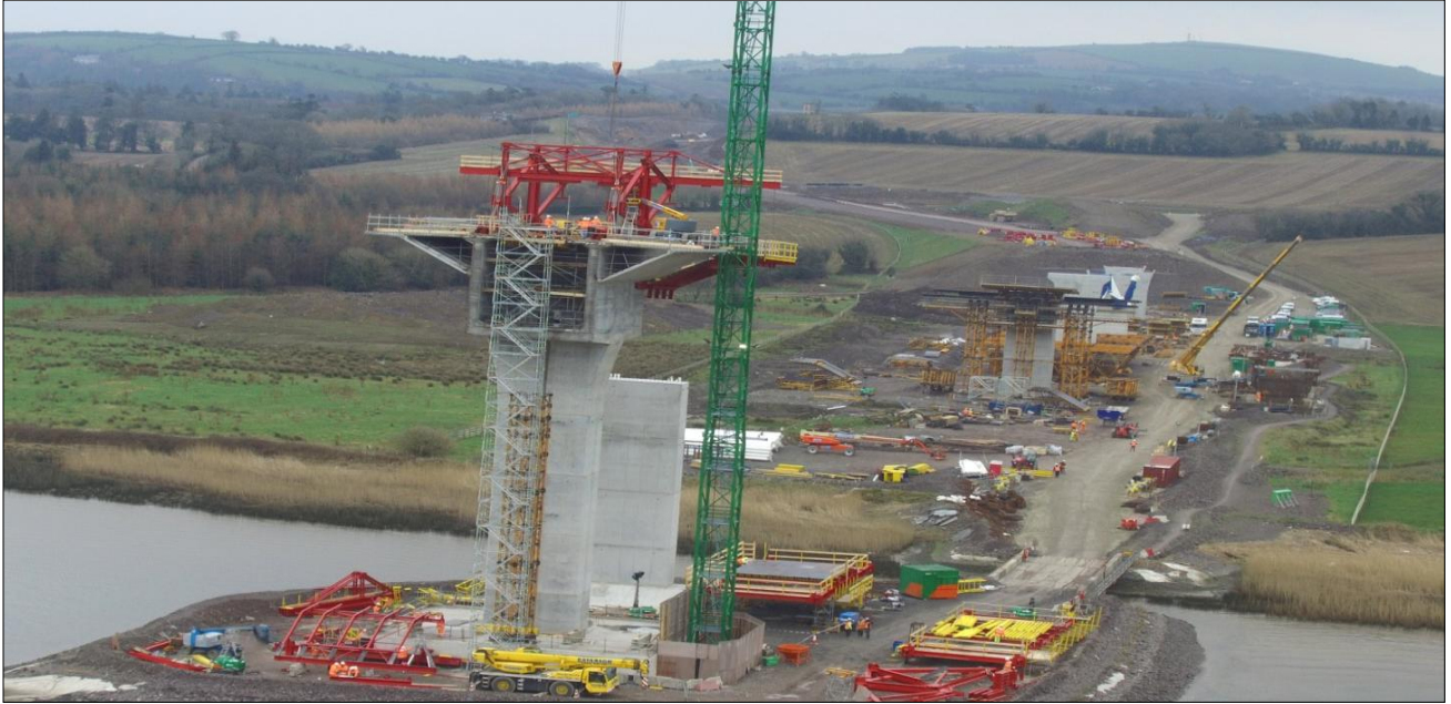
5. Barrow Bridge – Form traveller system assembled on top of pier 4 deck section in preparation for construction of deck on main spans. Temporary support pier visible immediately behind pier 4. Piers 5, 6, 7 & 8 in background.
