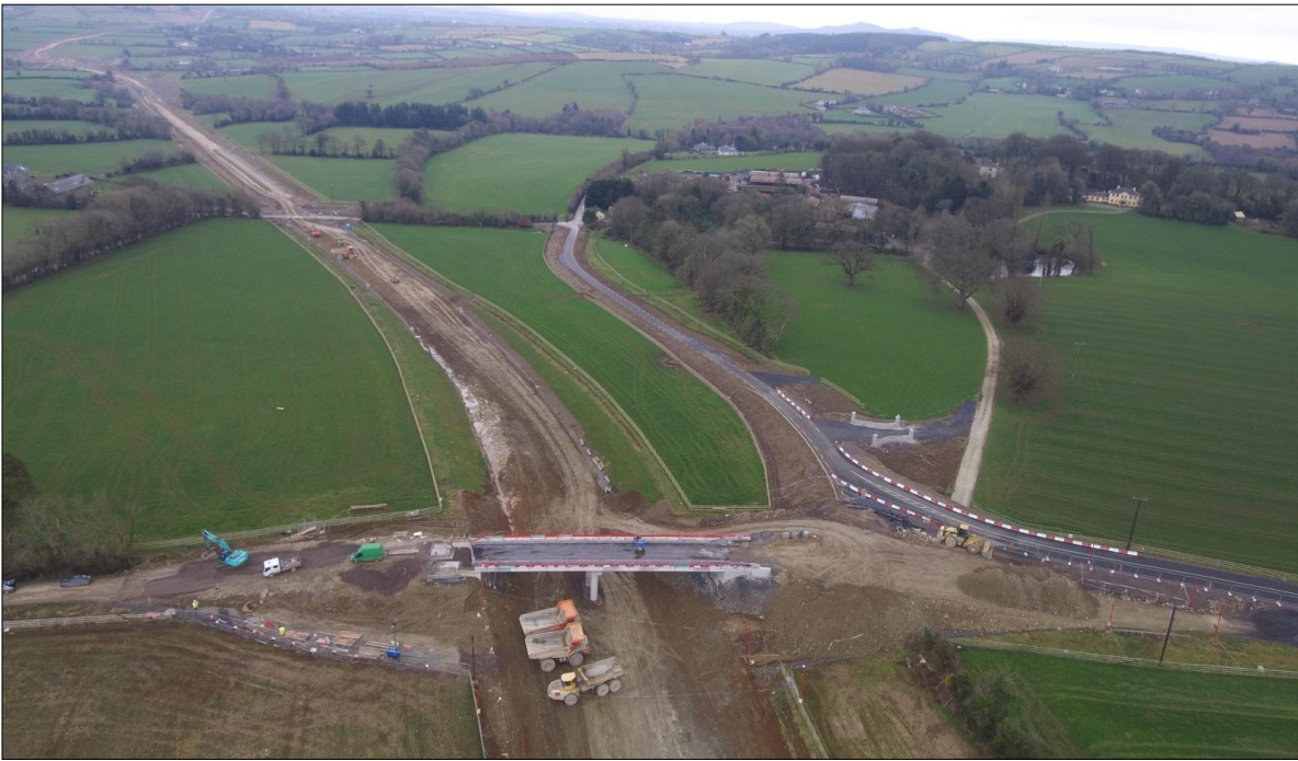
7. L-8142 Arnestown Road closed in foreground for construction of overbridge. Temporary diversion route via newly constructed L-8045 Road visible to the right. Road due to re-open after Easter. Newly constructed entrance walls (accommodation works) visible to the right of the diversion route.
