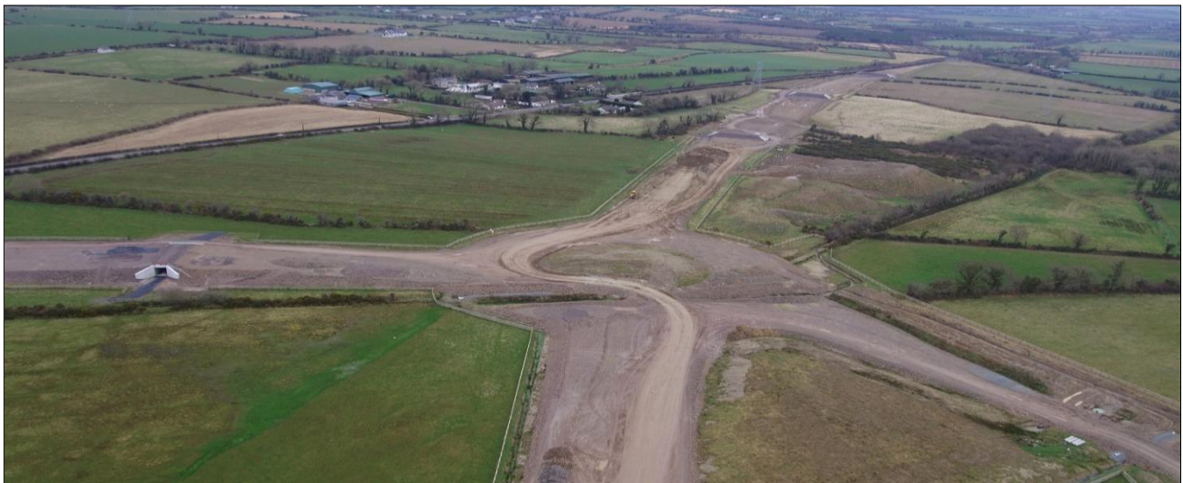
8. N30 Corcoran's Cross Roundabout under construction. Note farm underpass to the left of the roundabout and three further underpasses in the distance heading towards the N30 Enniscorthy.
