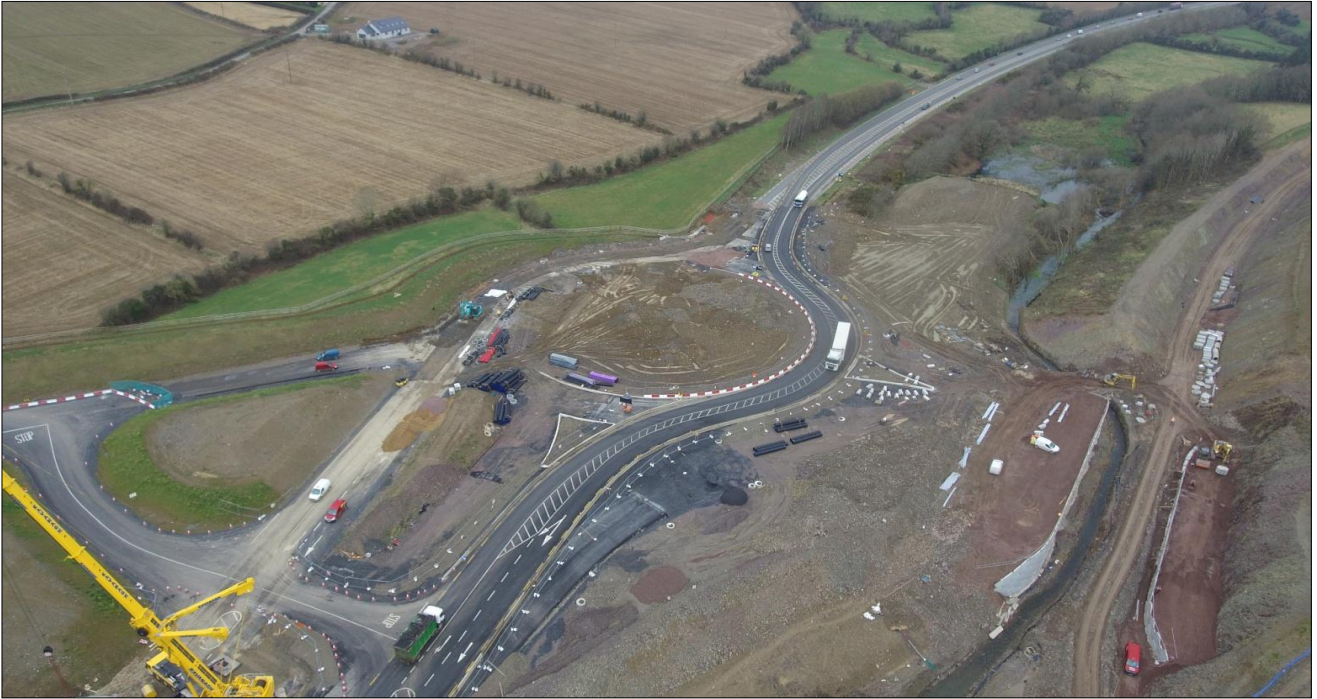
1. Temporary traffic management through Glenmore Roundabout. Works continuing on opposite side of roundabout in preparation for full opening in May. Construction of new Ballyverneen Road Overbridge and realignment visible to right of photo.
