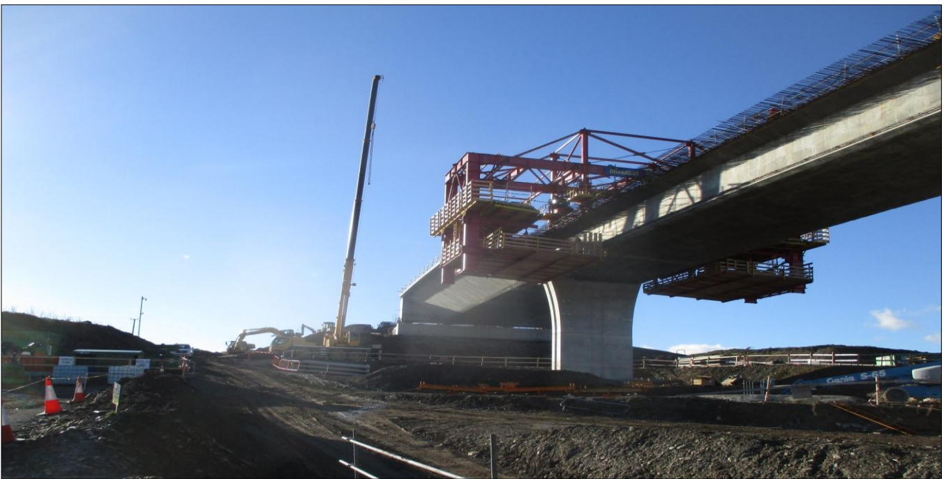
4. Barrow Bridge – wing traveller system set up on span 2, completed deck edge section visible on span 1 behind.
