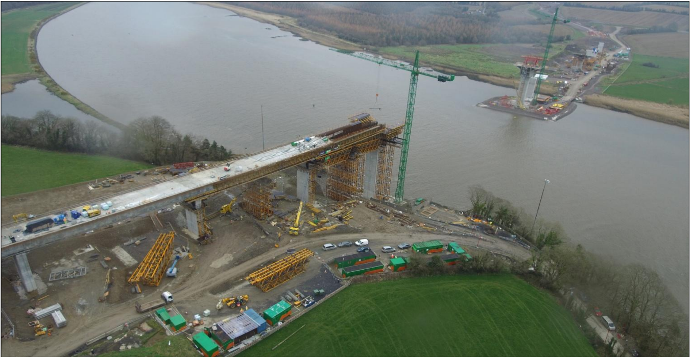
3. Barrow Bridge – Span 3 (near side) progressing to pier 3 with falsework partially still in place, pier 4 visible on far side.
