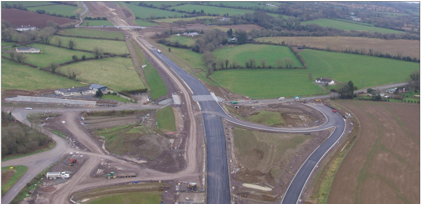
6. R733 Junction – Pavement works progressing on mainline and slip roads, R733 continuing to operate under mainline. Camlin Road Overbridge and realignment visible in background
