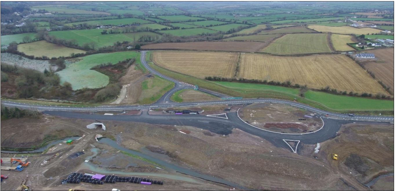
1. Works at Glenmore Roundabout for next phase of traffic management and completion of road underpass.
