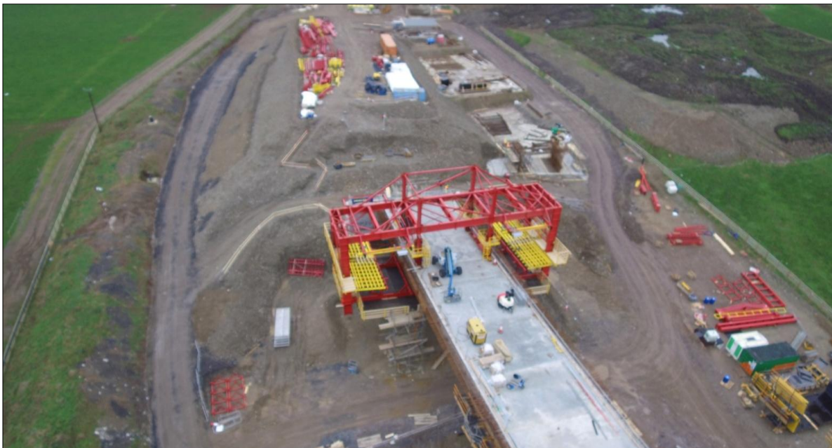
4. Barrow Bridge – Wing traveller assembled at span 1.
