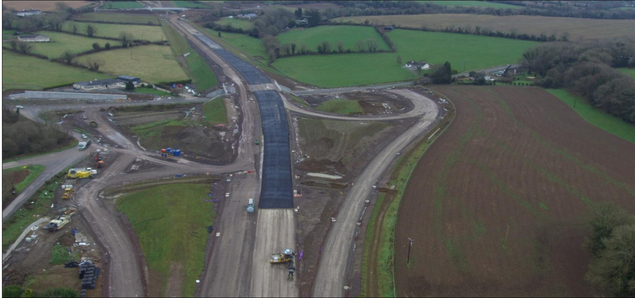
5. R733 Grade Separated Junction taking shape, and Upper Base laid on mainline.
