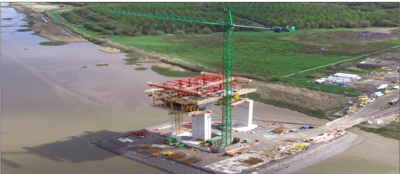
3. Barrow Bridge – Pier 4 and temporary pier from above
