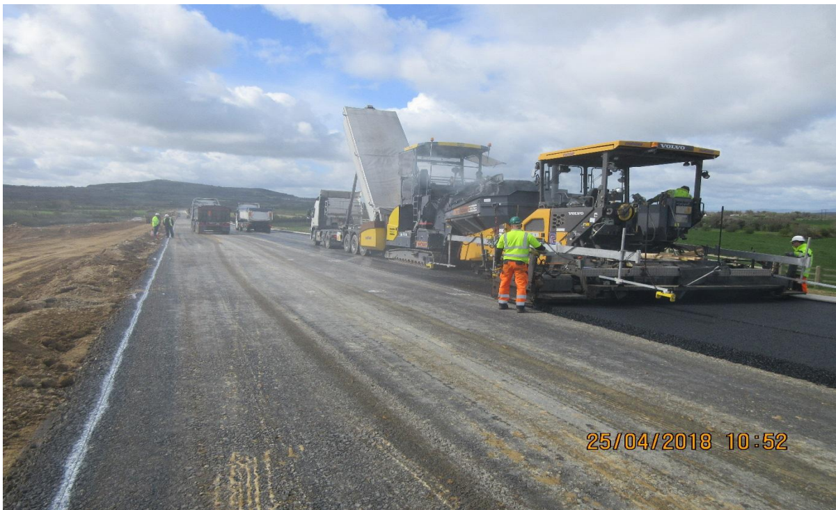
Laying Base Course on CBGM on M11 Northbound Carriageway
