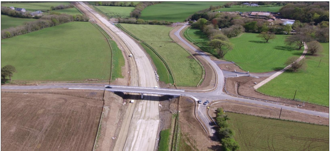
6. R733 Grade Separated Junction – pavement works under construction.
