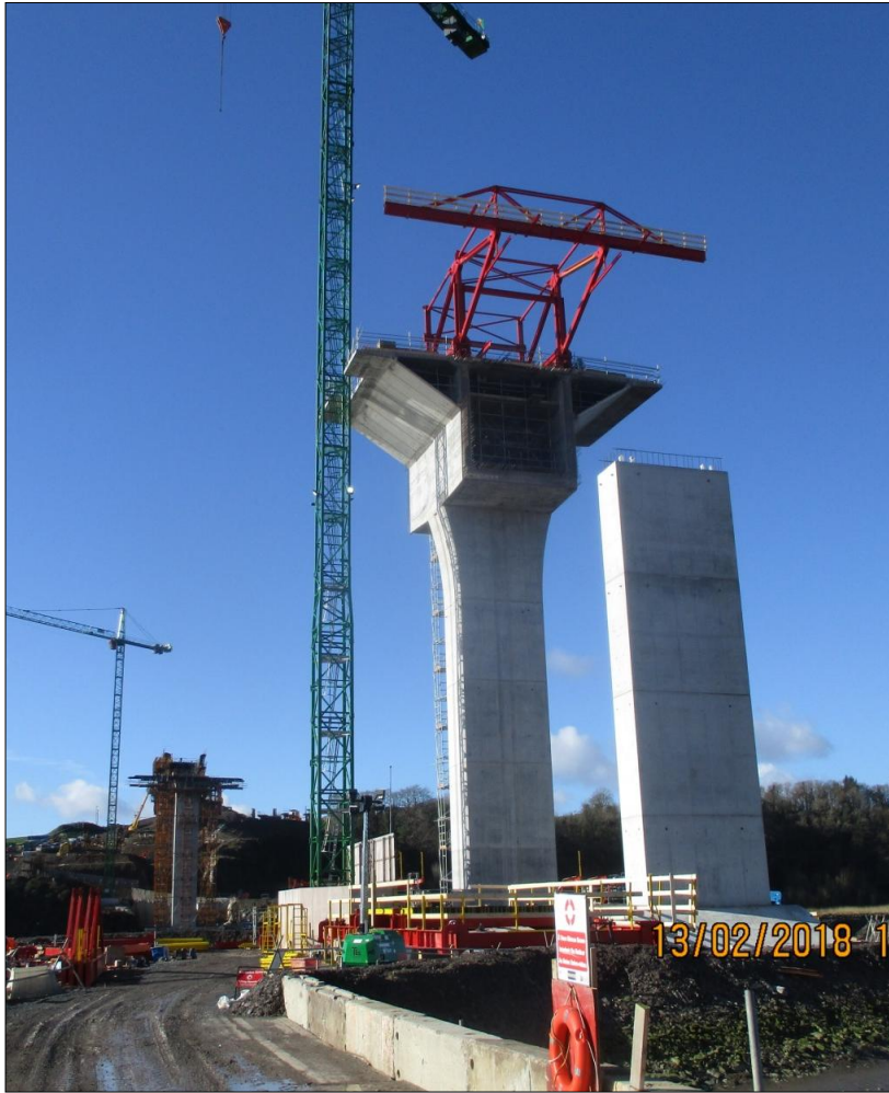
3. Barrow Bridge – Pier head for Pier 4 complete with form traveller under assembly. Temporary pier in front of pier 4.
