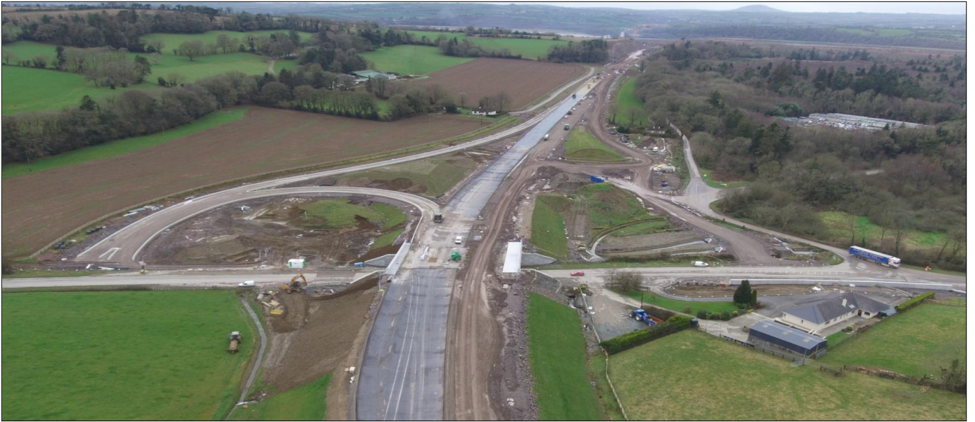
5. R733 Junction – Pavement foundations and kerbing on slip roads and blacktop on mainline (R733 running under mainline).
