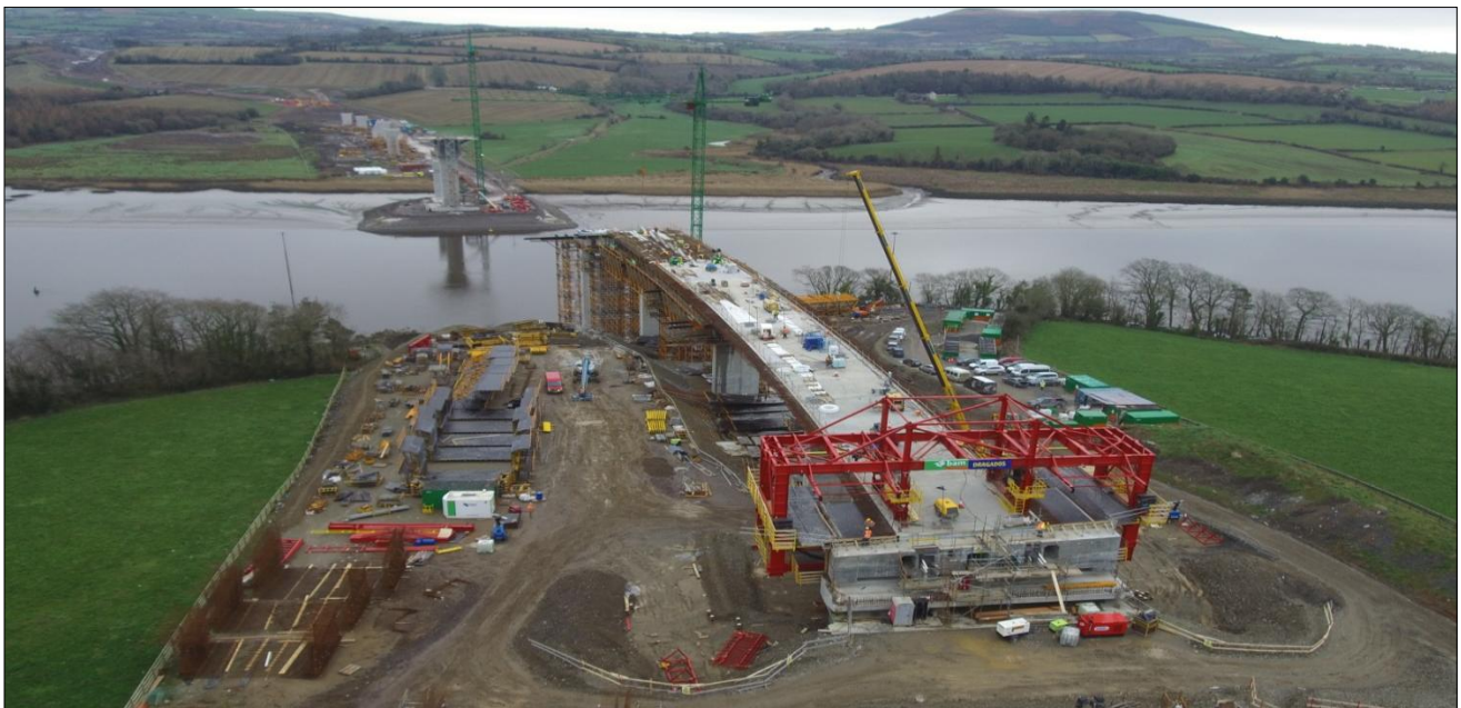
2. Barrow Bridge at Pink Rock – central deck complete for spans 1 & 2 in foreground with wing traveller in place for construction of deck edge sections. Support falsework still in place for span 3.
