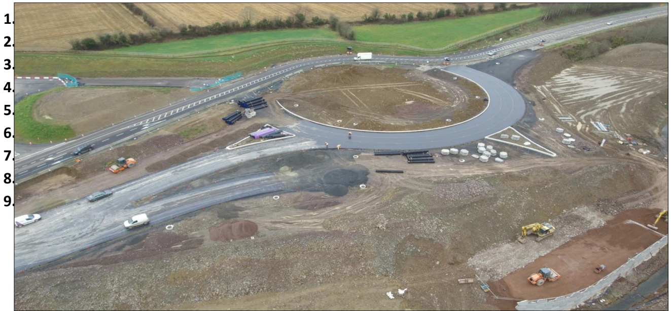
1. Pavement and kerbing works for next phase of traffic management at Glenmore Roundabout (now open to traffic).
