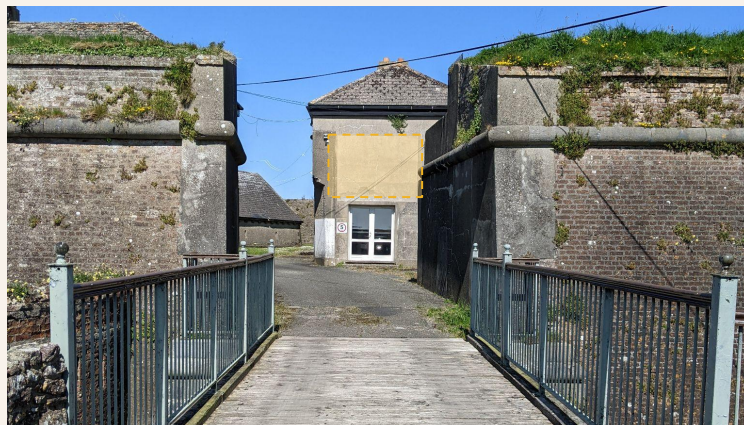
View of current shared vehicular and pedestrian entrance into the Fort over the bridge
