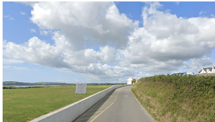
Section of road-side parking with no footway along Strand Road 'R737' (Source: Google Maps)
