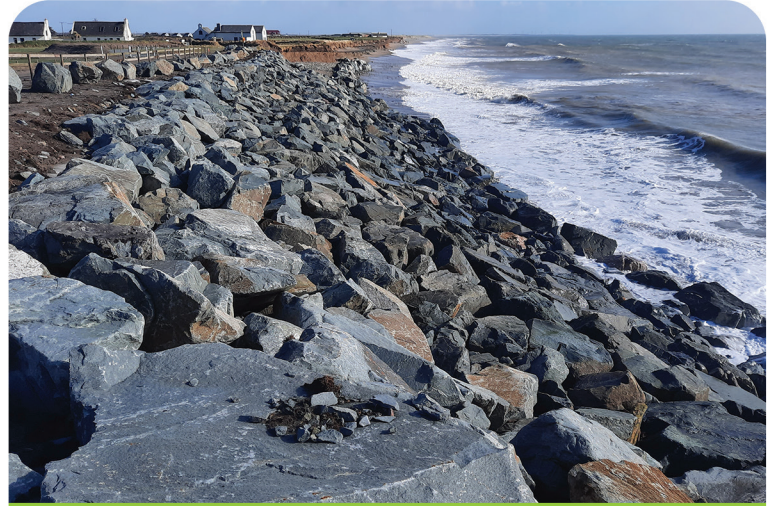
Seaview Coastal Protection Works
