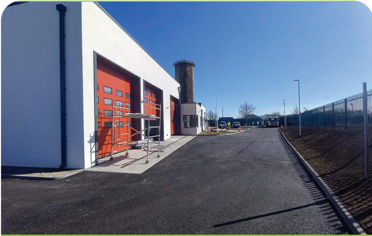
New Fire Station, New Ross
