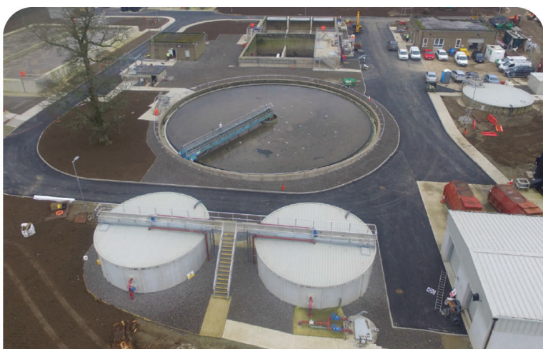
Upgrade of Enniscorthy Waste Water Treatment Plant
