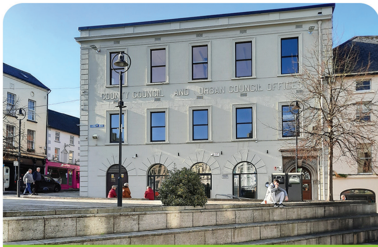
Enniscorthy Courthouse & Municipal District Office Redevelopments
