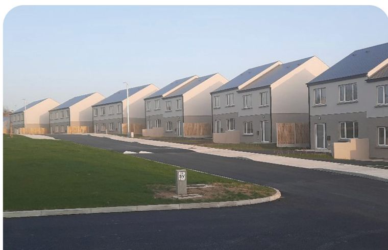
Carley's Bridge Housing Scheme
