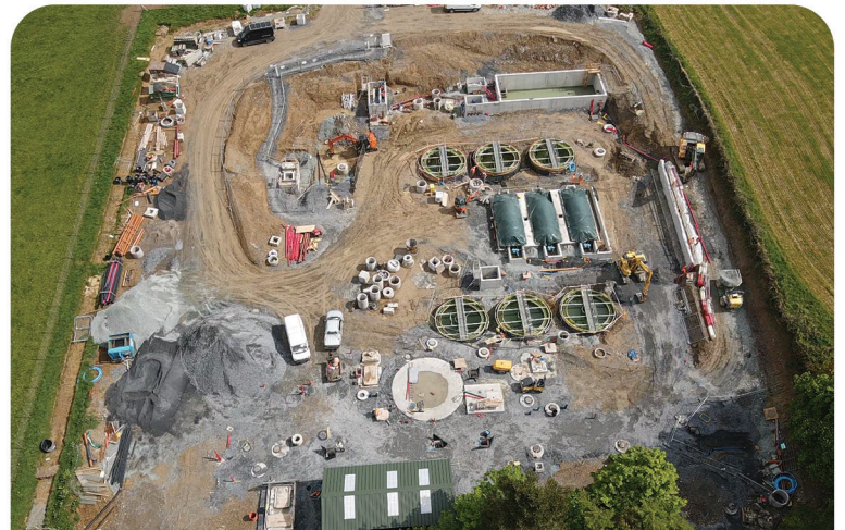
Duncannon, Arthurstown and Ballyhack Waste Water Treatment Plant
