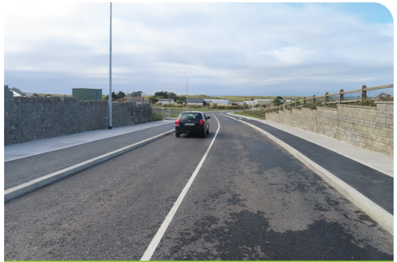
Kilmore Quay Link Road
