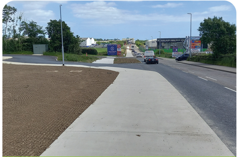
Wexford Town Active Travel Improvements
