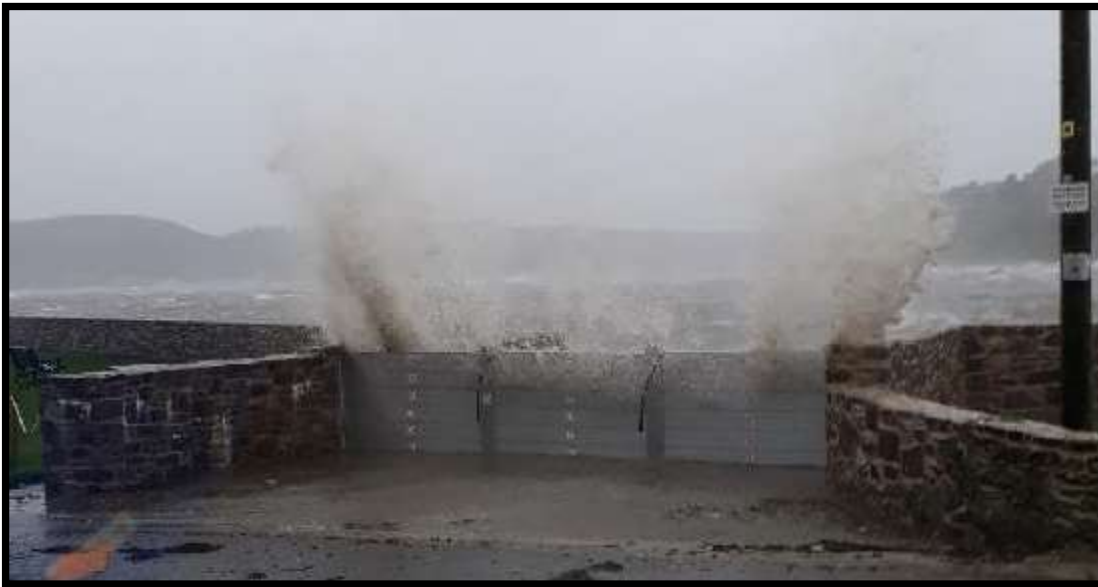
Arthurstown – Storm tides on the 16/10/17 (new demountable barrier during storm tides)
