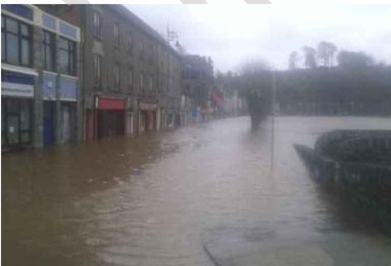
Shannon Quay Flooding (12:07pm)
