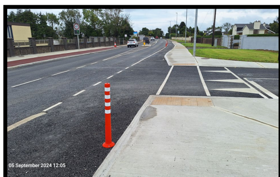
Completed phase 1 Newtown Rd Works, Maldron Roundabout in foreground with bus shelters and segregated cycling lanes.
