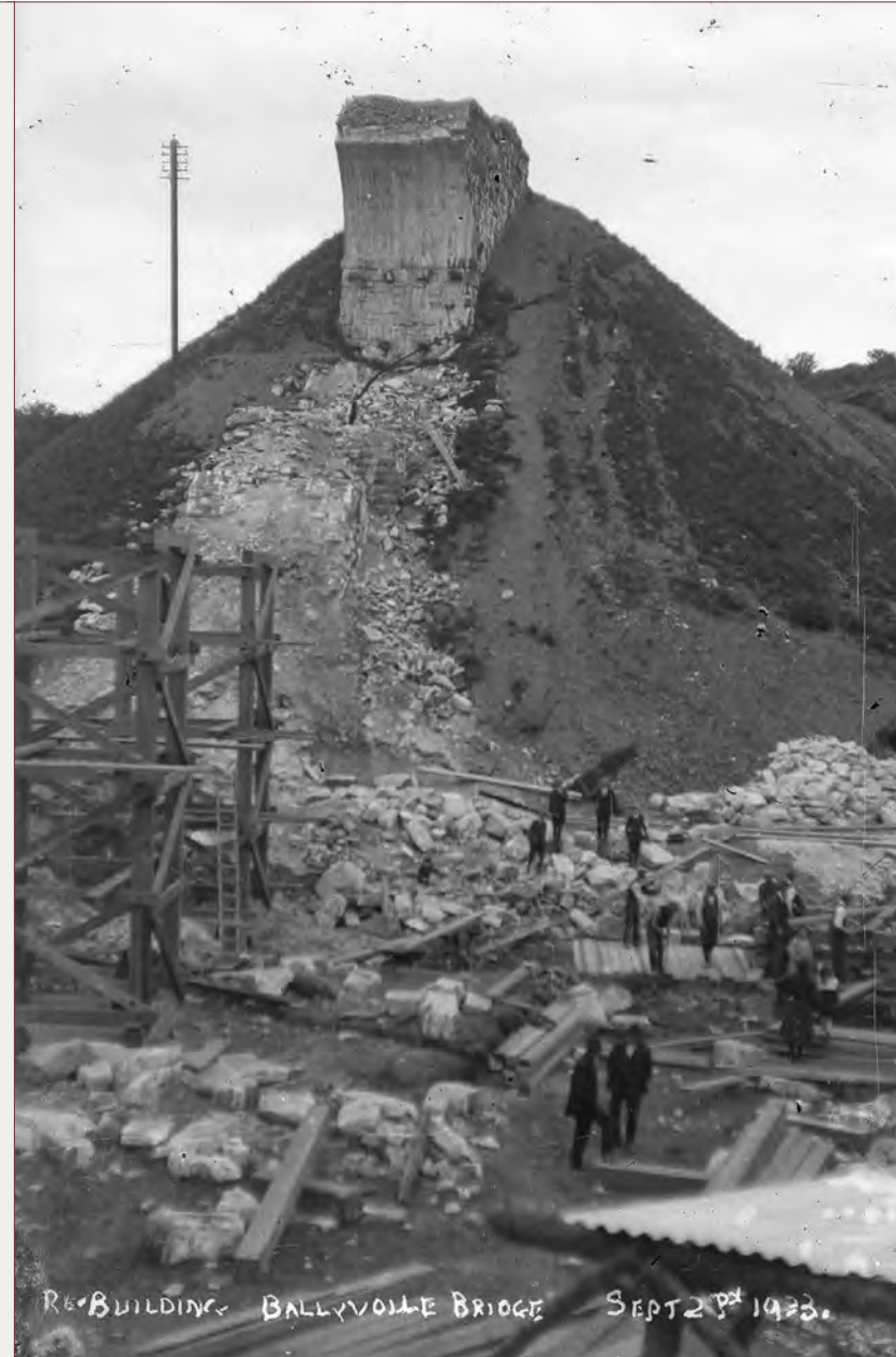
Rebuilding Ballyvoyle Railway Viaduct, Waterford. Courtesy of Waterford County Museum, EK 273.
