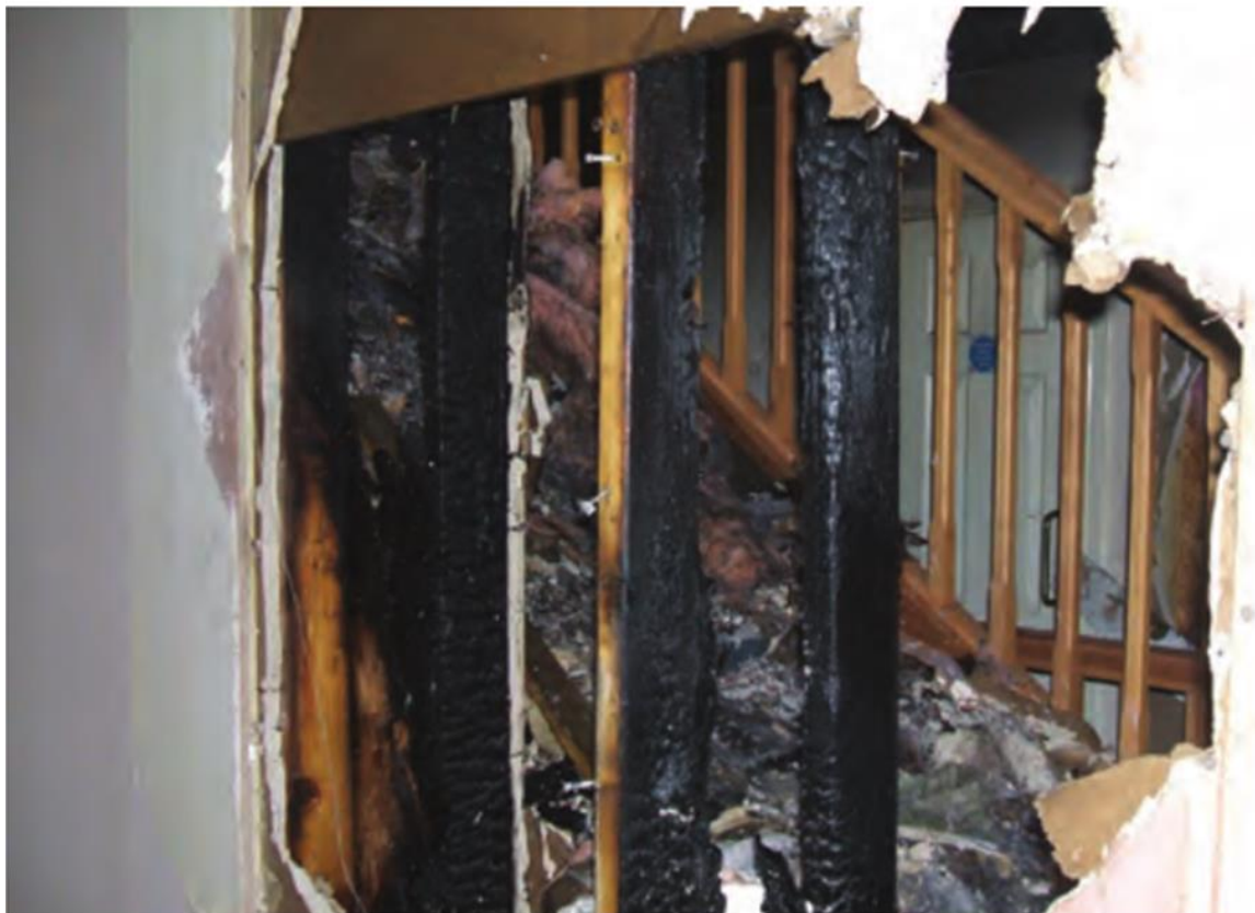
Back to Back penetrations in stud partition
