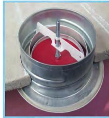
Fire Rated Ceiling Air Valve installed before a fire
