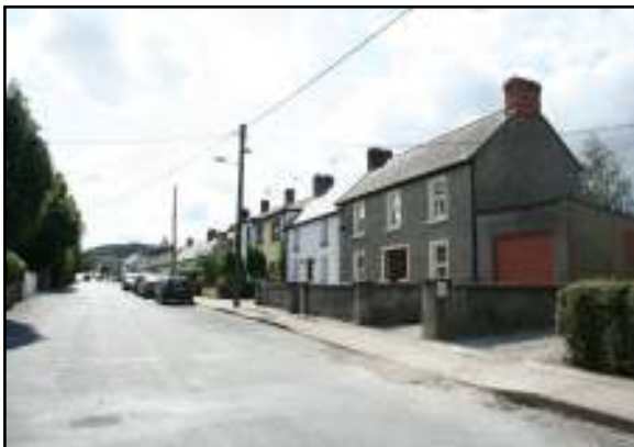
Above: Original terraced buildings on Church Street.
