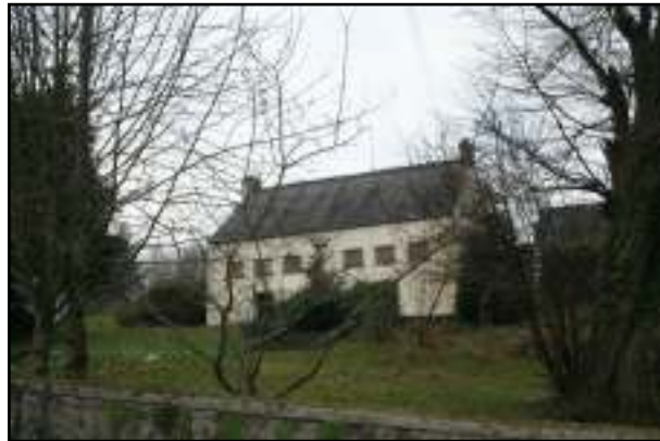
Above: Vacant Old School Building on Hospital Hill
