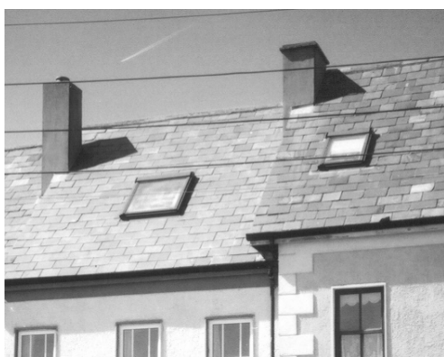
Plate 3.2 Suitable roof lights
