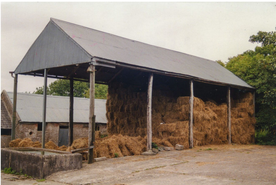
Hay barn of vernacular character, with timber pole supports and pitched roof, near Barringtonsbridge, Co. Limerick (Barry O'Reilly)
