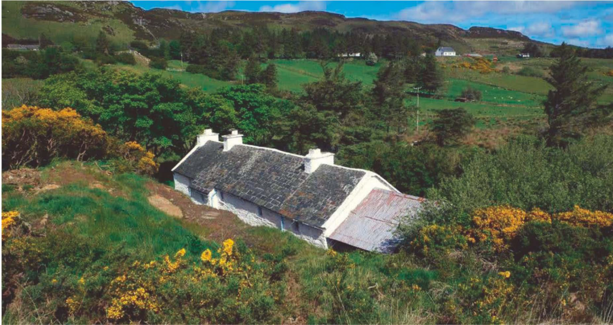
House with Roshine Slate roof, taking full advantage of the shelter of the slope, near Dunfanaghy, Co. Donegal (Joe Gallagher/Greg Stevenson)
