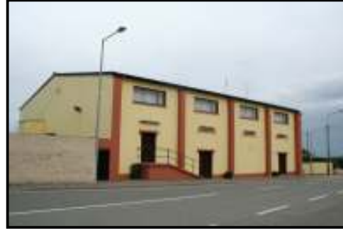
Above: Clonroche Community Centre
