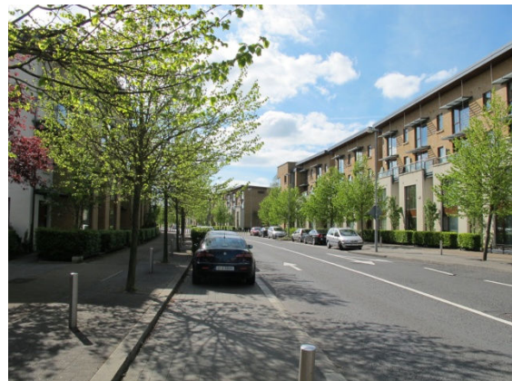
Photo 2 An Avenue with three storey frontage
