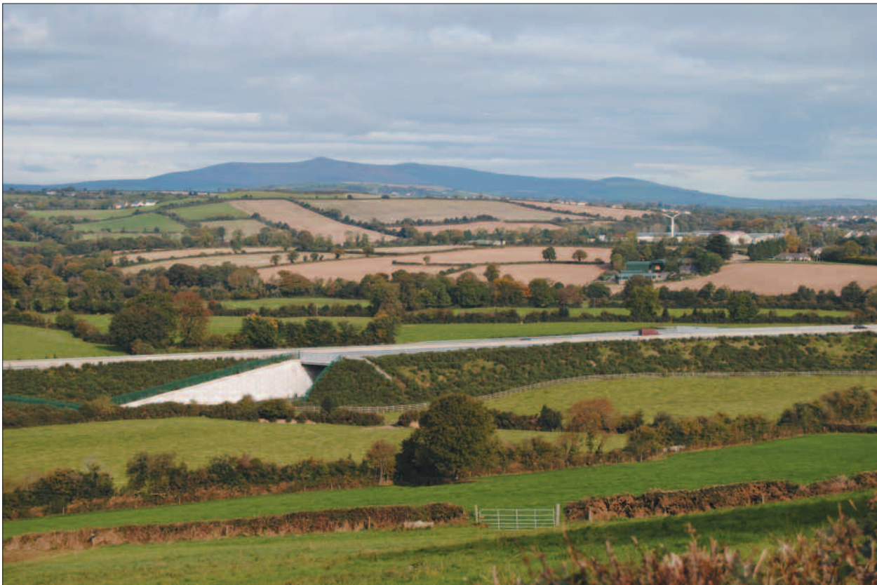
Above: Section of the M11 Gorey bypass.
