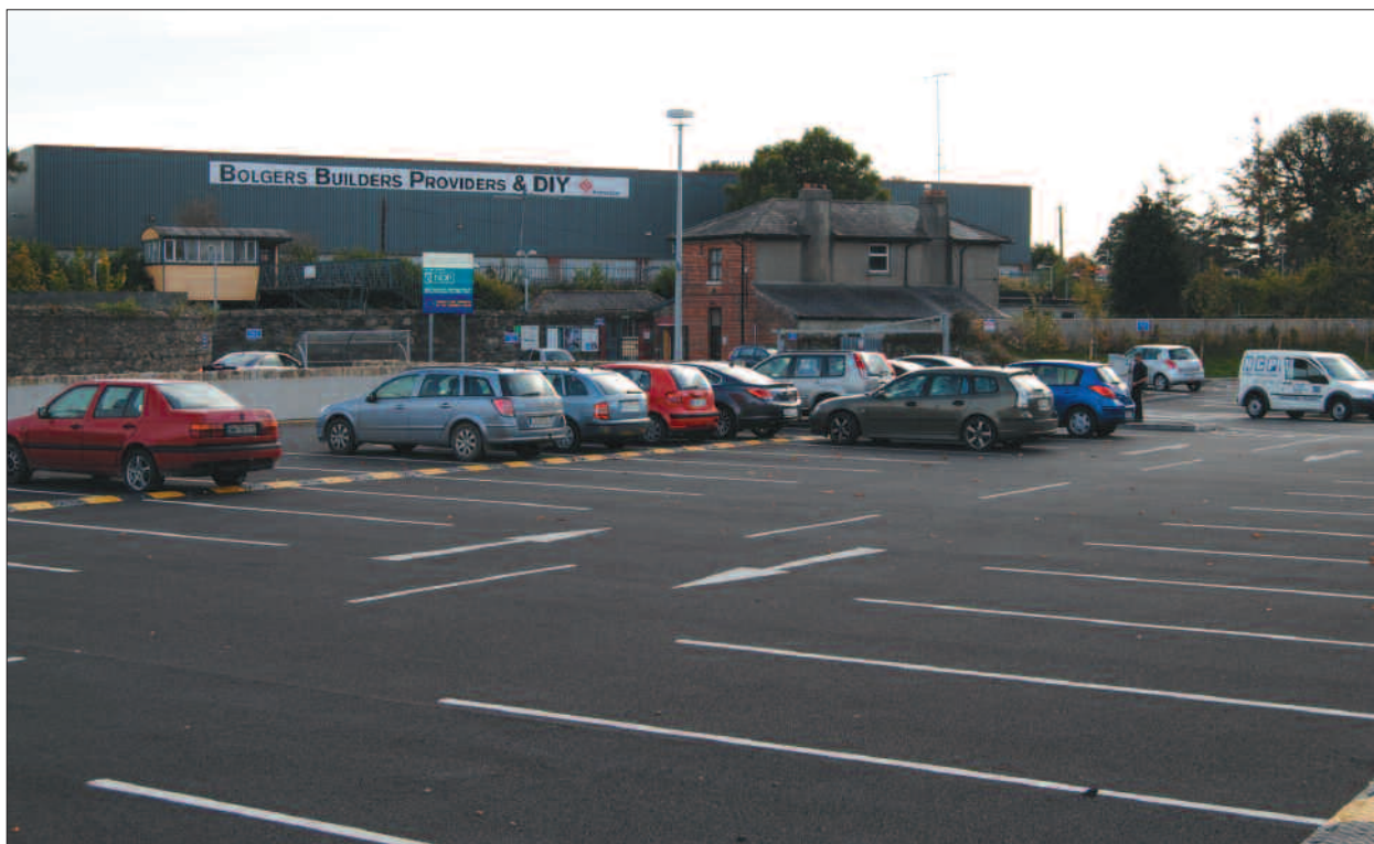
Above: New car park at Gorey Train Station.
