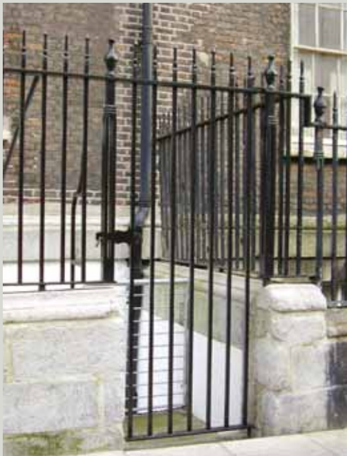
This replacement gate has been inserted sensitively and has been designed to tie in with the proportions and design of the original railings
