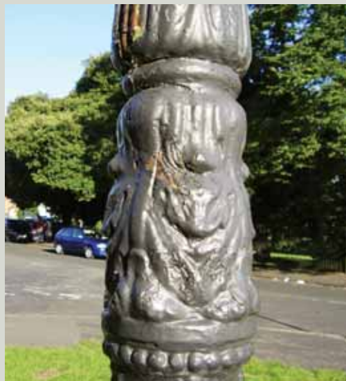
Over-thick application of paint will obscure detail and result in less effective protection
