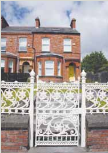
Cast iron railings and gate, Limerick
