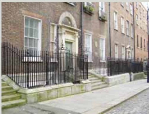
Early eighteenth-century wrought iron railings, Henrietta Street, Dublin. The large-scale development of squares and terraces from the 1700s onwards fuelled a rising demand for iron railings
