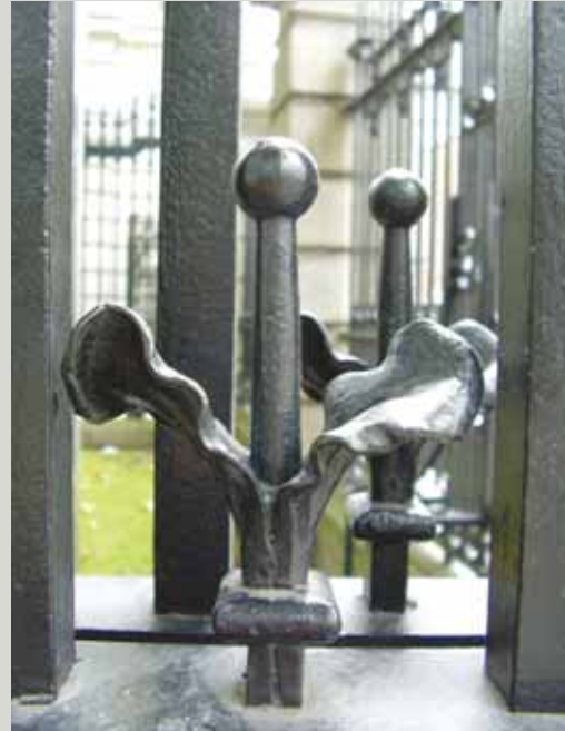
A new section of gate, based on the design of the adjacent gate at the entrance to Leinster House, Dublin. To prevent corrosion, water traps should be filled so that they shed water, or pinholes drilled at the base to allow water to escape (although drilling into original fabric should be avoided where possible)
