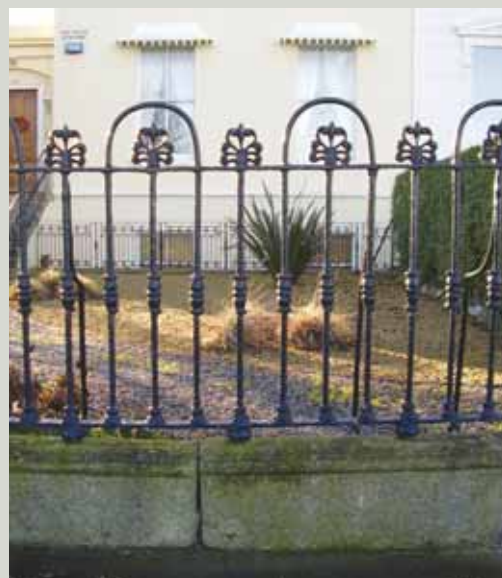
Early nineteenth-century railings incorporating fashionable Neo-Classical decoration such as cast iron collars, husks, and anthemion (honeysuckle) finials
