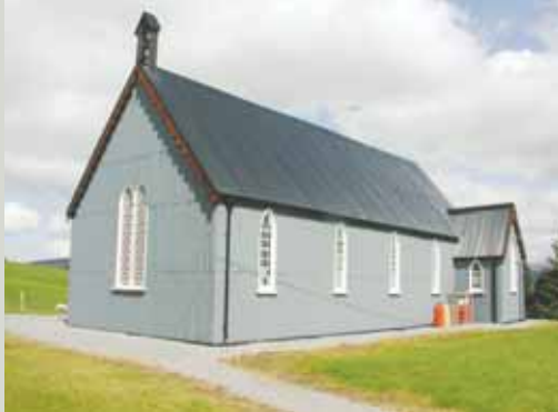
Lurganboy Church of Ireland church, County Leitrim. A fine example of a corrugated-iron clad 'tin church' built in 1862
