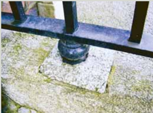
A stone indent has been inserted to repair a fracture or widened socket
