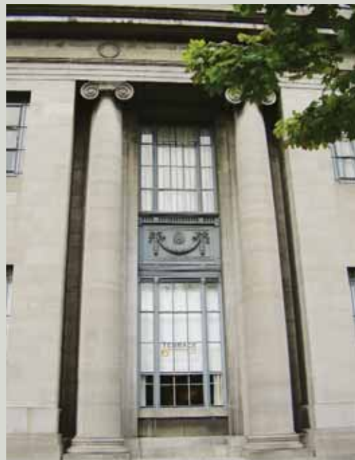
The National Concert Hall, Earlsfort Terrace, Dublin. Cast iron windows and spandrel panels became increasingly widespread from the start of the twentieth century. This example was supplied by the Scottish firm Walter Macfarlane & Co. Ltd in 1914
