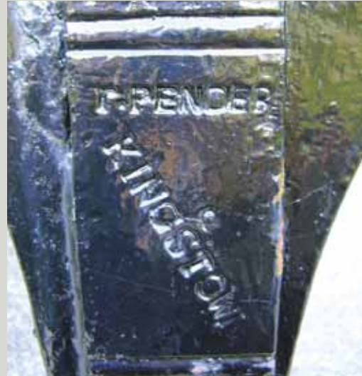
Blacksmiths often stamped their name on the flat slam bar (or cover plate) of gates
