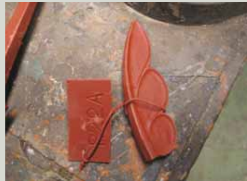
Attaching metal tags to ironwork as it is dismantled (numbered to correspond with a measured survey drawing) is essential for tracking repairs and for correct reinstatement (Image courtesy of Historic Scotland)
