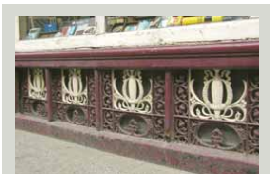
Routine maintenance to ironwork, such as this attractive cast iron stall riser to a shopfront should include gentle washing using a minimum amount of water to remove accumulated dirt
