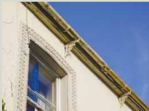
Cast iron gutter brackets, typical of the second half of the nineteenth century
