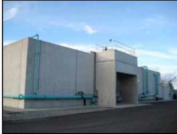
Above: Wastewater Treatment Plant Marshmeadows
