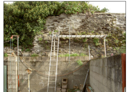
Ad hoc repairs to town wall in yard to south of 12 Abbey View
