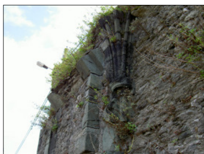
Surviving carved limestone arch and rib vault springing
