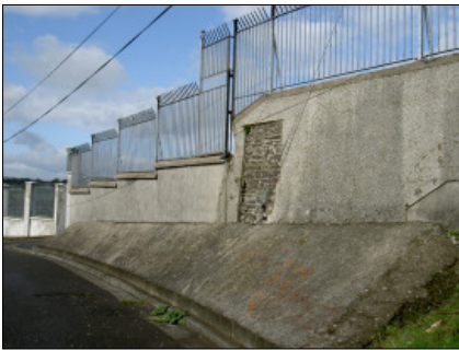
Rubble stone panels in school boundary wall
