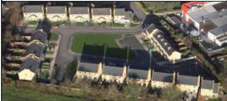
Ariel view of Castle Court in Taghmon
