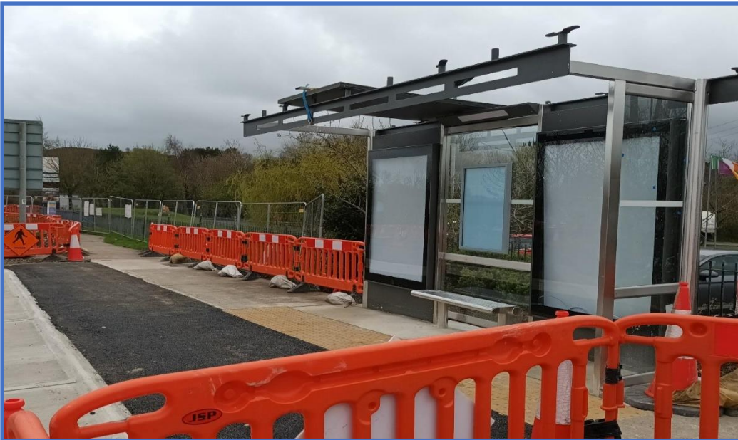
New bus shelter erected outside Maldron Hotel on Newtown Road
