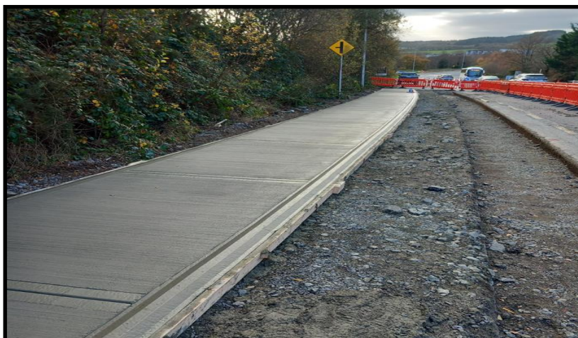
New footpaths with delineator kerb and sub base of new cycle paths at Newtown Road
