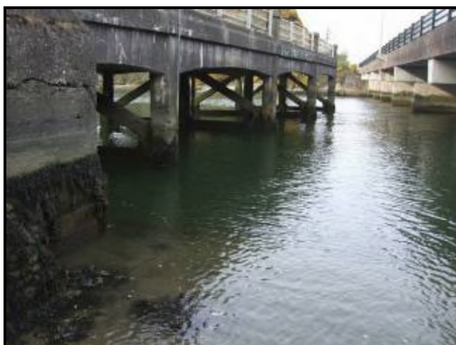
Plate 9 Ferrycarrig Bridge at the proposed crossing points C1 and C1A on the Slaney estuary during low tide.
