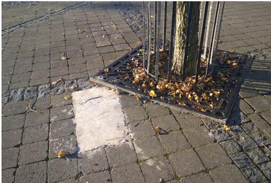
4. Commercial Quay: Patch Repairs to paving in alternative materials
