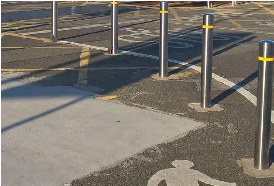
8. Paul Quay: Surface patching over pedestrian lining/delineation
